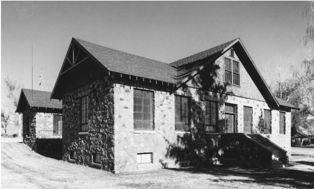
Stewart Indian School, to the south of Carson City, was one of a few off-reservation federal schools built for Native Americans. The campus includes dozens of historic buildings, most of which were built by students learning how to become masons.
