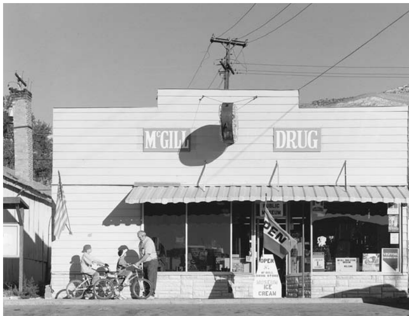
The McGill Drugstore building dates to as early as 1909. The institution served as a pharmacy for the company town until 1979.
