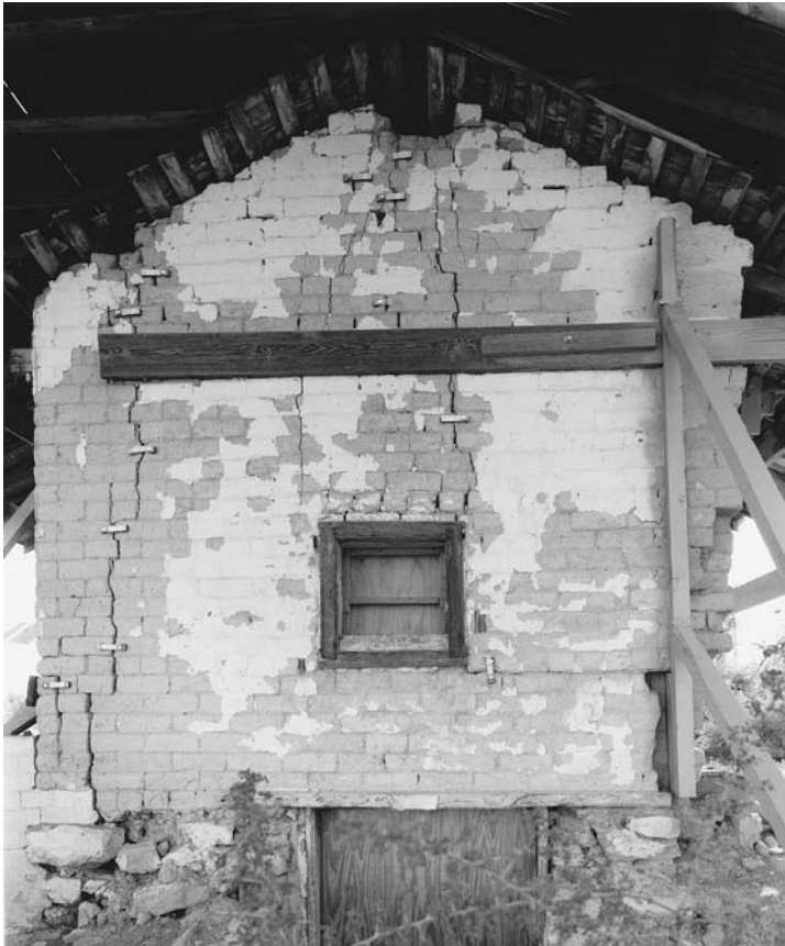
The adobe walls of the Kiel Ranch are showing stress and will not last much longer without a great deal of assistance.
