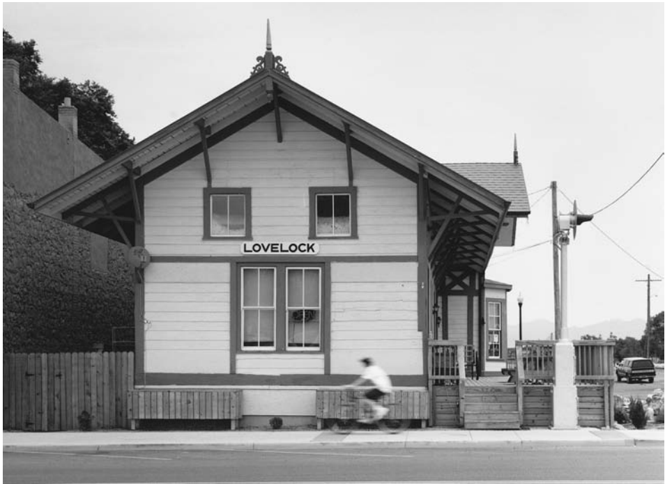
Lovelock's railroad depot, completed in 1880, is an excellent expression of Eastlake-style design.
