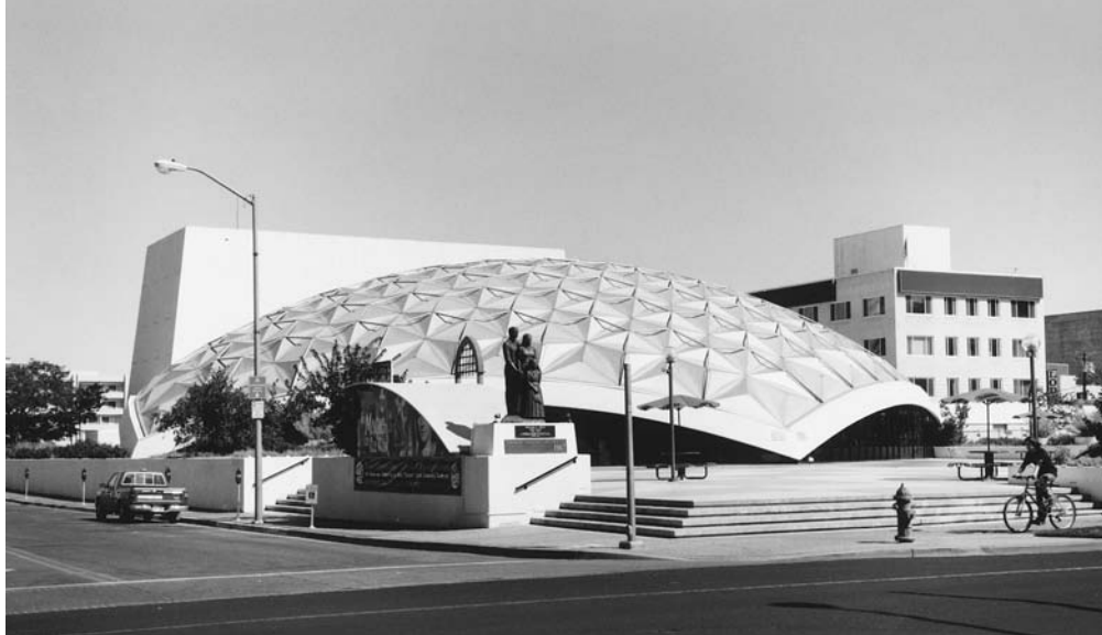
The Pioneer Theater-Auditorium, completed in Reno in 1967, features a striking metal geodesic dome.
