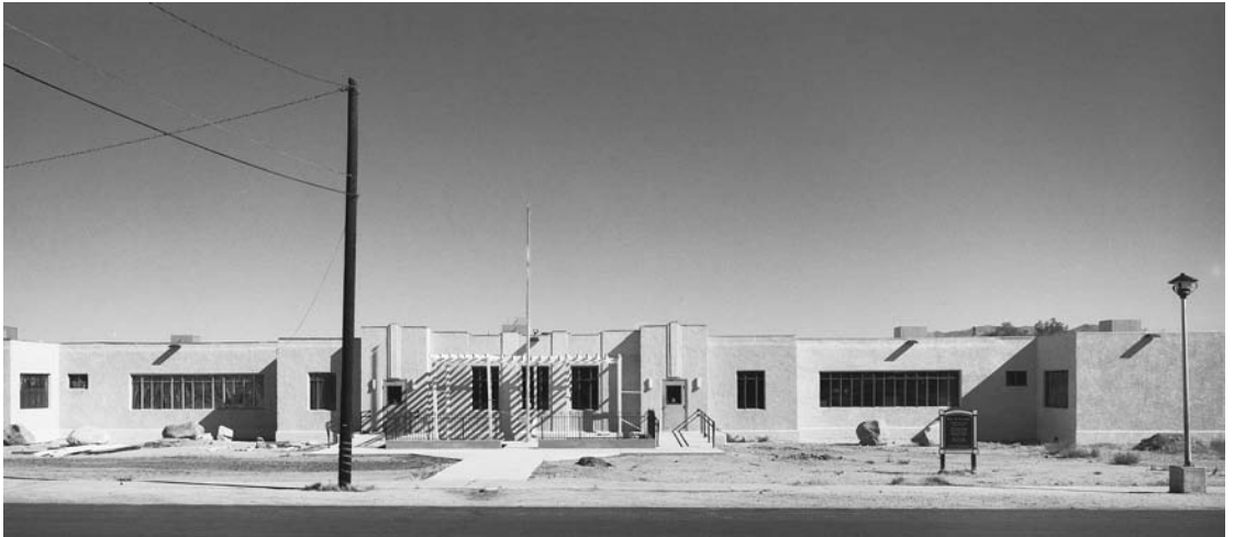
Hawthorne built its Sixth Street School with federal funds from the Public Works Administration, a New Deal program in the 1930s. After 1997, the facility became an arts center.
