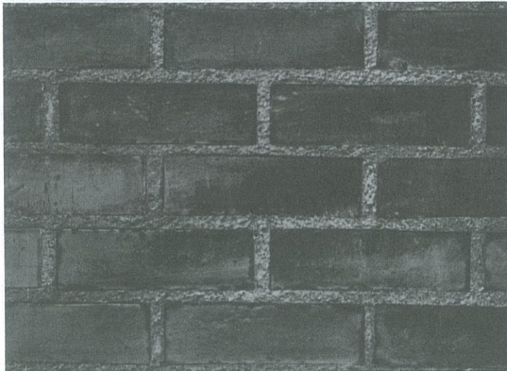
Figure 24. Flush-cut joints, sack-rubbed.
