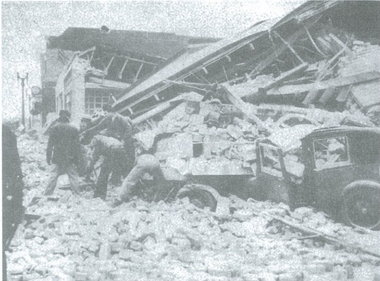
Unreinforced masonry building after 1933 Long Beach, CA earthquake.
