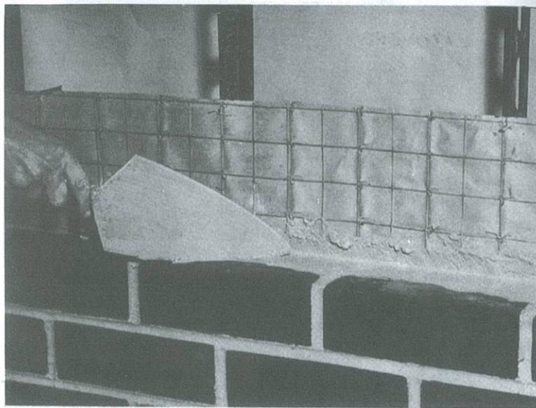
Figure 35. "Steeltex" tied to steel studs, being slush grouted.
