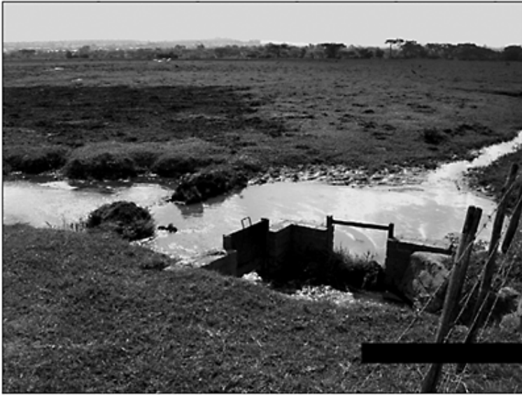
Figure 9.4. Crowborough pasture – a distribution chamber for SEM.
