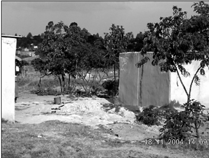
Figure 6.5. Shallow well (on left) in close proximity to a pit latrine (on right).
