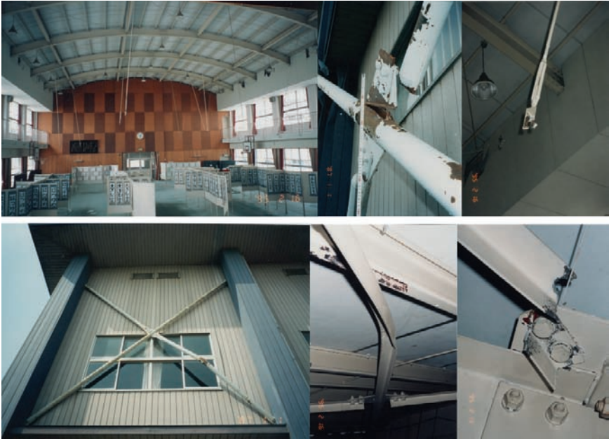
Fig. 9-10. Braces in steel frames
