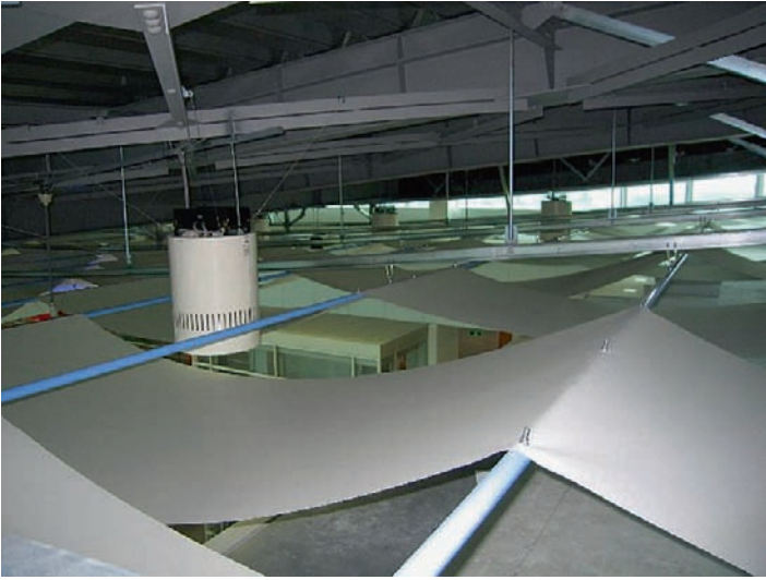
Fig. 9-40. Details of the membrane ceilings
