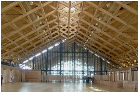
(1) Heavy Timber Structure
