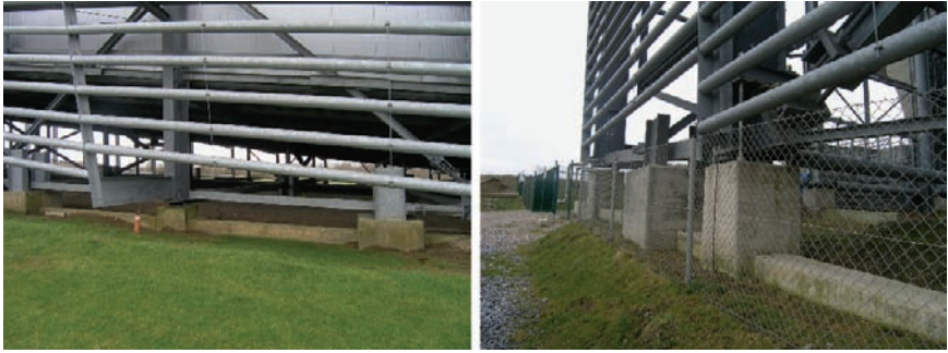
Fig. 14-27. Big footing foundation upon former landfill
