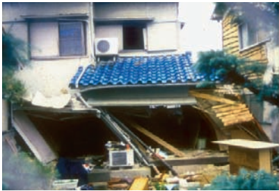
Fig. 10-7. Lack of wall
