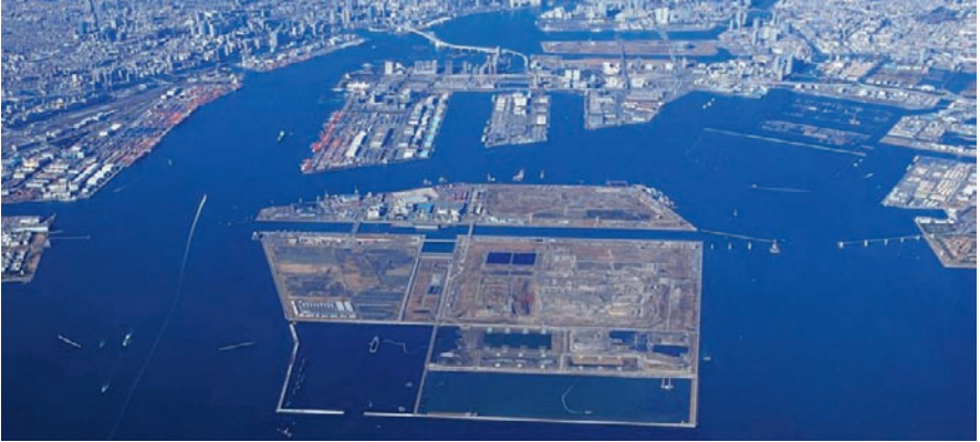
Fig. 14-11. Municipal waste island in Tokyo harbor area in operation (©Bureau of Port and Harbor, Tokyo Metropolitan Government)
