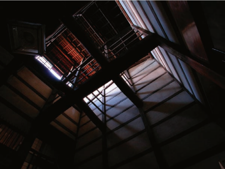
Fig. 5-6. Skylight of townhouse in Joetsu
