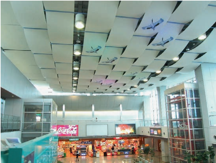
Fig. 9-39. Membrane textile ceilings in the reopened Kushiro airport
