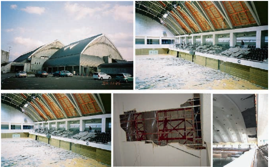
Fig. 9-29. Damage to ceiling systems in public halls in Nagaoka city
