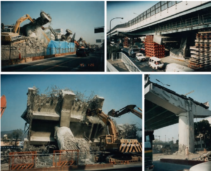
Fig. 9-7. A highway supported by cantilever columns
