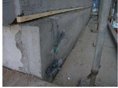
Reinforcement of Existing Foundation
