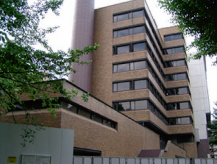
Fig. 8-18. Building No.11 of school of engineering (before seismic rehabilitation)
