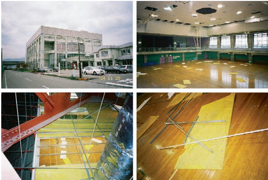
Fig. 9-28. Glass-wool ceiling panels in a public gymnasium in Nagaoka city
