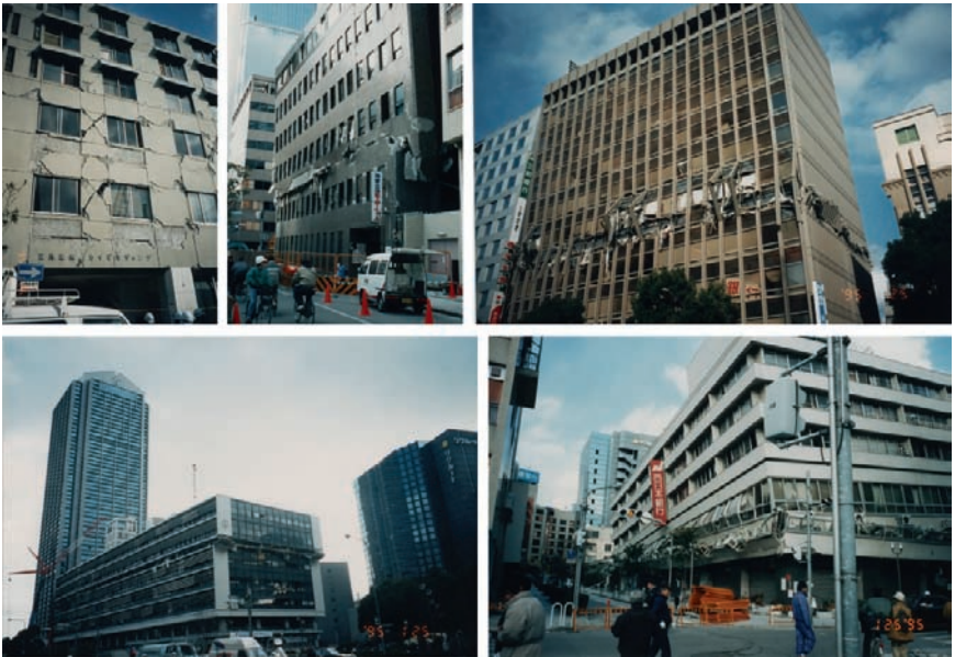
Fig. 9-6. Middle-story buildings damaged by Kobe earthquake
