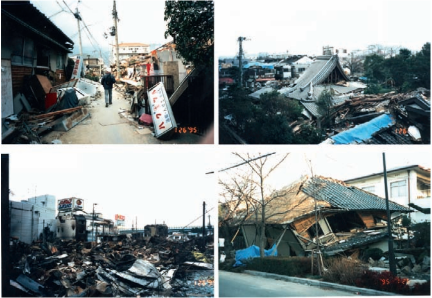
Fig. 9-5. Wooden houses damaged by Kobe earthquake
