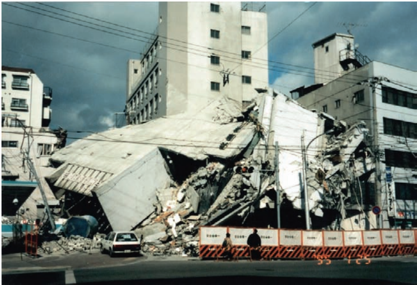
Fig. 9-3. A completely collapsed reinforced concrete building
