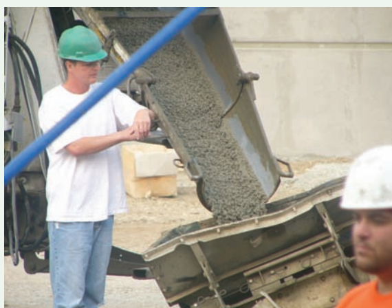
Figure 3-18 Pervious concrete discharging into the belt-placer (telebelt) hopper, Lacey, WA
