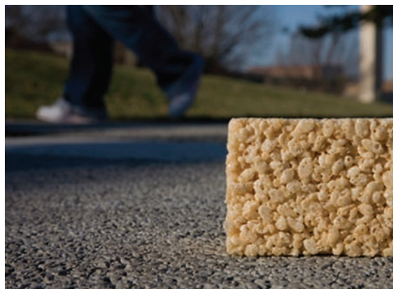
Figure 3-2 Typical pervious concrete surface, Kansas City, MO Source: University of Missouri-Kansas City
