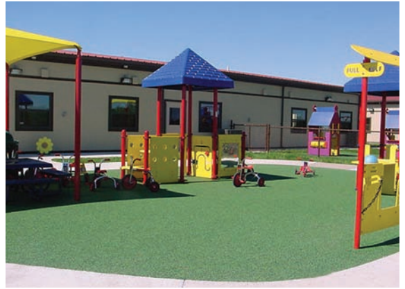
Figure 3-11 Completed playground with artificial grass over pervious concrete, Fort Riley, KS Source: Concrete Promotional Group, Inc.
