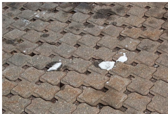
Figure 8-19 A stain remover applied to PICP is ideally allowed to set overnight.
