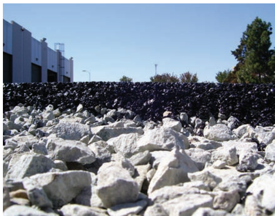
Figure 2-11 Porous asphalt section, San Diego County Operations Center, CA
