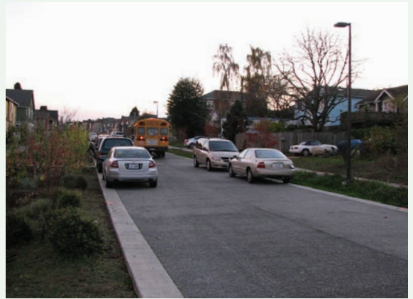
Pervious concrete in Seattle, WA Source: Amy Rowe
