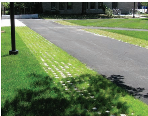
Figure 1-1 Castellated concrete grid pavement at walkway edges, Cambridge, MA
