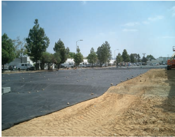
Figure 2-16 Earthen berms and geotextile, San Diego, CA
