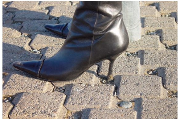
Figure 8-15 PICP openings and joints must be filled with aggregate to prevent tripping hazards. Source: NCSU
