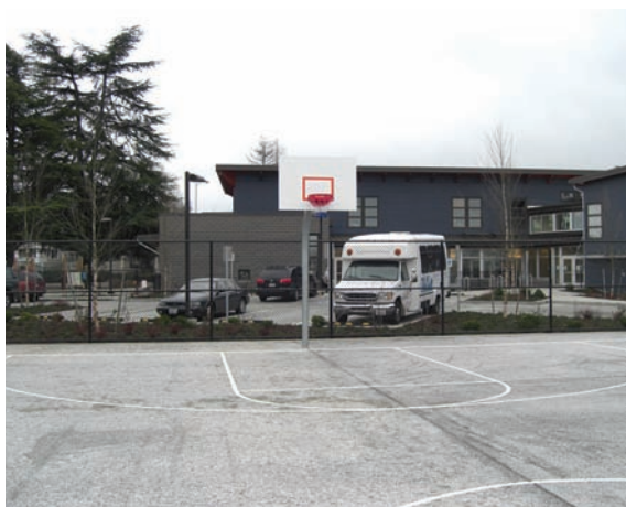
Figure 7-2 Pervious concrete basketball court provides infiltration and sound absorption for local residents, Neighborhood House Community Center, Seattle, WA
