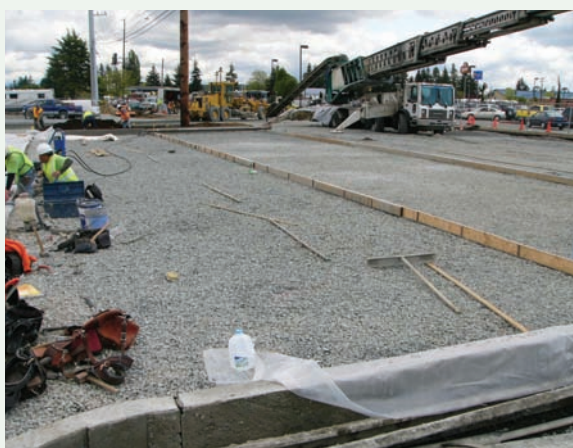
Figure 3-17 Forms and tools in place before concrete arrives, Seattle, WA
