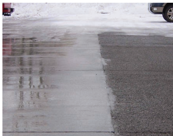
Figure 1-2 Standard concrete pavement (left) next to pervious concrete (right) during winter, Iowa State University, Ames, IA
