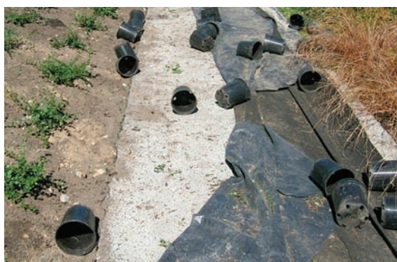
Figure 7-7 Protective covering prematurely removed from pervious concrete sidewalk, resulting in clogging Source: SvR Design Company
