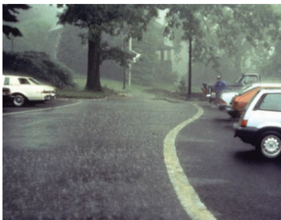
Figure 2-4 Parking lot with standard aisle and porous asphalt stalls, Morris Arboretum, Philadelphia, PA Source: CH2M HILL
