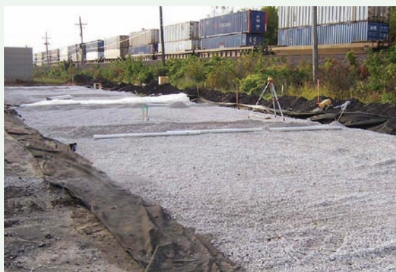
Figure 3-16 Aggregate base after installation of geotextile fabric, Ames, IA
