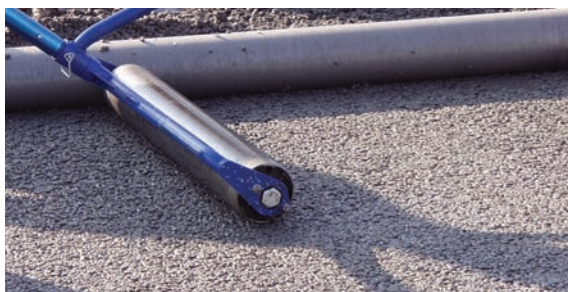
Figure 6-8 Example of pervious concrete installation with an added sorbative admixture
