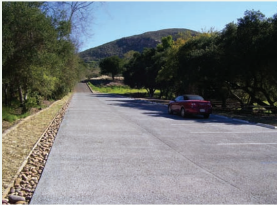
Pervious concrete in San Diego County, CA Source: CH2M HILL
