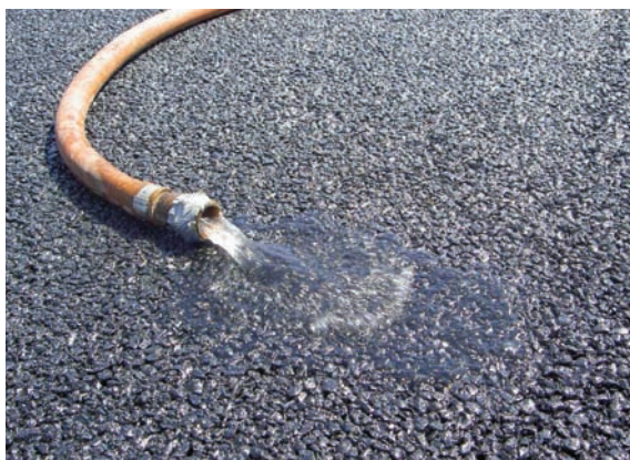
Figure 2-2 Porous asphalt surface at Port of Portland, OR Source: Century West Engineering
