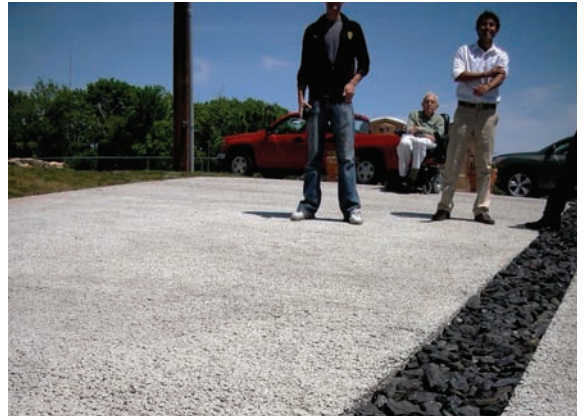
Figure 3-7 Pervious concrete residential driveway, Kansas City, MO Source: John Kevern
