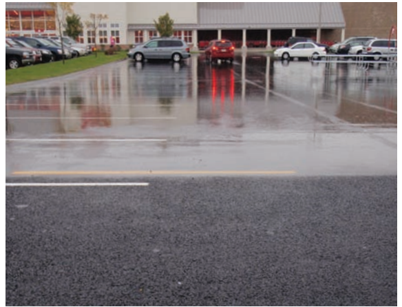
Figure 2-6 Commercial parking lot with standard pavement and porous asphalt, Greenland Meadows, Greenland, NH
