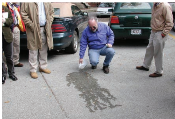
Figure 8-7 Demonstration of clogged pervious concrete surface using one gallon of water, Savannah, Georgia
