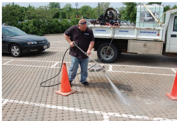
Figure 8-20 Subsequent pressure washing of PICP after the stain remover has set
