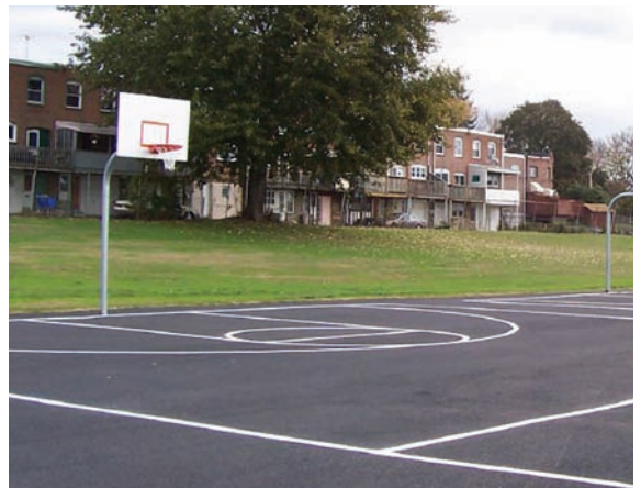
Figure 2-8 Porous asphalt basketball court, Upper Darby, PA
