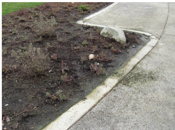
Figure 7-6 Sediment from unstabilized soils flowing to permeable pavements, Neighborhood House Community Center, Seattle, WA
