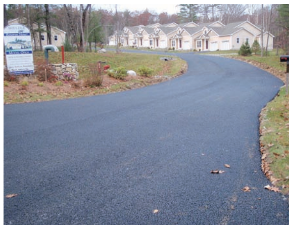
Figure 2-3 Porous asphalt residential lane, Pelham, NH Source: Rosen, R. M.
