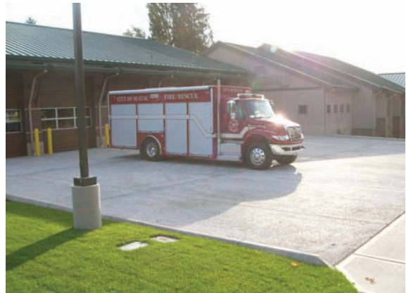
Figure 3-13 Pervious concrete at a Fire Station, SeaTac, WA Source: Puget Sound Concrete Specification Council
