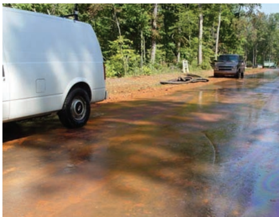
Figure 8-2 Nearby construction increases the risk of sedimentation of permeable pavement Source: NCSU
