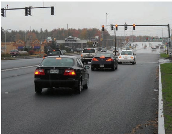
Figure 2-7 Permeable pavement test section on state highway using open-graded friction course over and asphalt treated permeable base (ATPB), MaineDOT, Portland, MA
