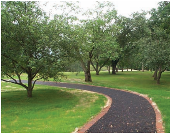
Figure 2-5 Porous asphalt path, Grey Towers National Historic Site, PA
