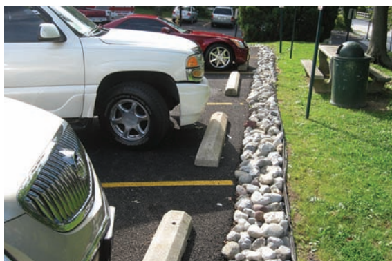
Figure 2-13 River stone edge offers a backup method for runoff to enter the reservoir course, Yeadon, PA
