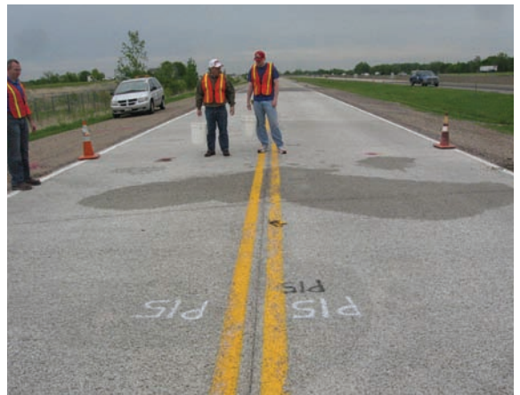
Figure 3-9 Pervious concrete overlay at a MnROAD Facility, Albertville, MN Source: John Kevern
