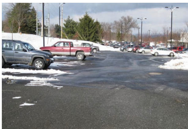
Figure 2-9 Dry porous asphalt in foreground and conventional pavement in the background, Cayuga Medical Center, Ithaca, NY
