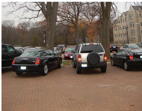
Figure 8-3 Leaf and tree detritus collects in PICP openings located underneath a tree line, Chicago, Illinois Source: NCSU
