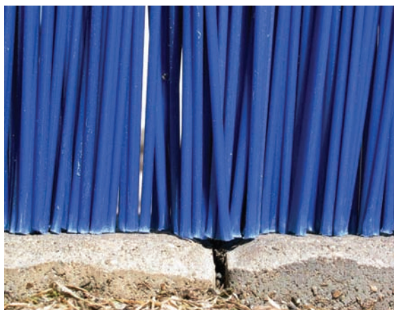
Figure 8-18 Pavement types with small openings or gaps (such as PICP) will not be easily reached by sweeper bristles.
