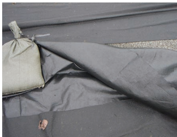
Figure 8-5 Tarp being used to protect pervious concrete from clogging, Seattle, WA Source: E. Fassman
