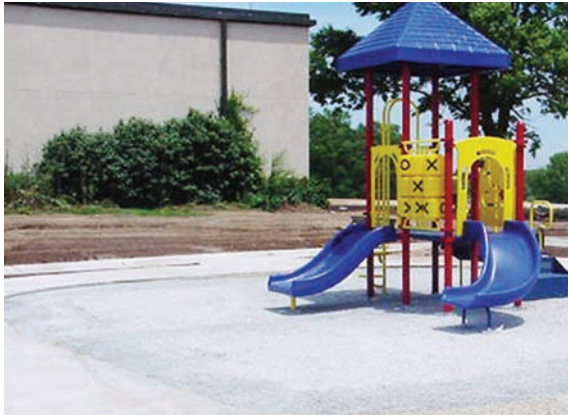
Figure 3-10 Pervious concrete as a drainage layer underneath playground, Fort Riley, KS Source: Concrete Promotional Group, Inc.
