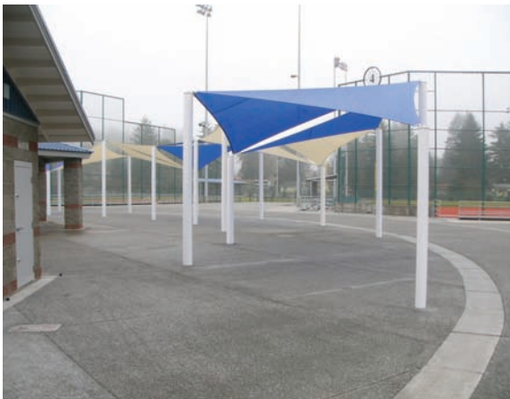
Figure 3-8 Pervious concrete at the Regional Athletic Complex, Lacey WA Source: Puget Sound Concrete Specification Council
