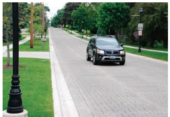
Figure 4-1 PICP roadway, Main Street, Warrenville, IL Source: ICPI
