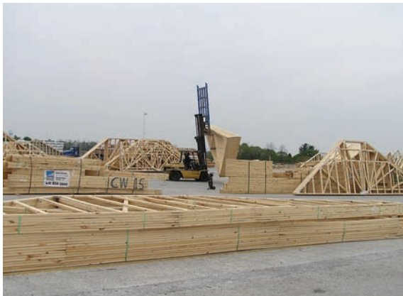
Figure 3-12 Pervious concrete on an industrial site, Shelter Systems, MD Source: National Ready Mix Concrete Association
