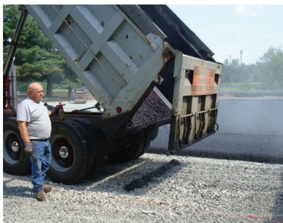
Figure 1-16 Installation of porous asphalt parking lot, North Shore MA Source: VHB
