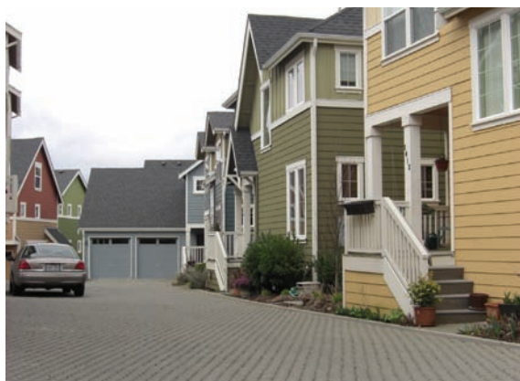
Figure 7-4 Permeable interlocking pavers serve as the drive access for multiple residences, Lyle Homes Development at High Point, Seattle, WA
