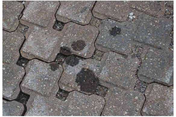
Figure 8-13 After vacuum cleaning of a PICP parking lot surface Source: ICPI
