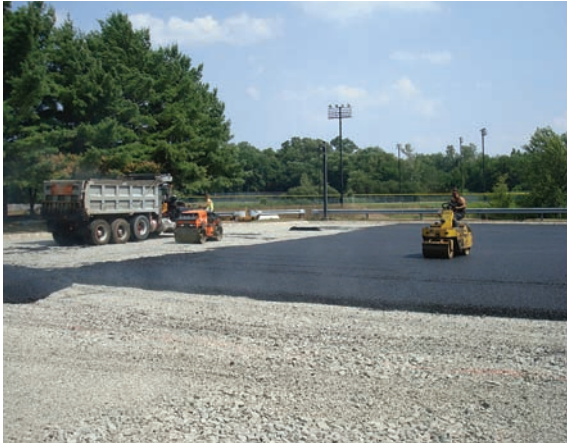
Figure 2-14 Porous asphalt installation, Peabody, MA
