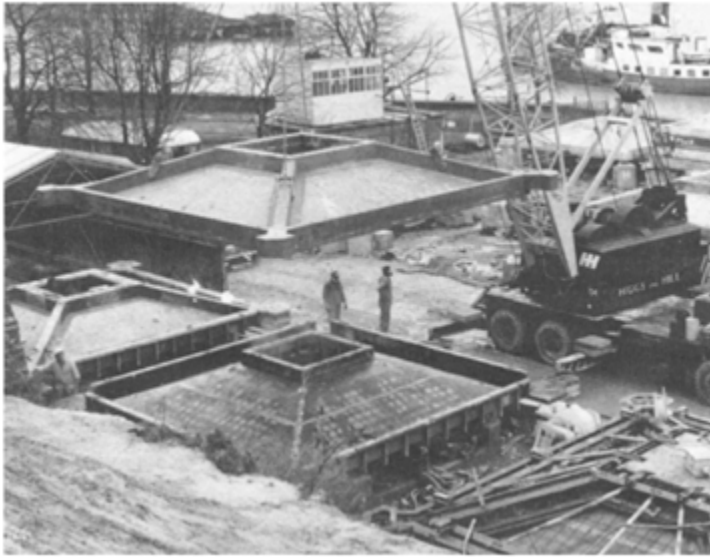
Demoulding a roof unit using mobile crane and specially fabricated lifting connections (Higgs and Hill Limited)
