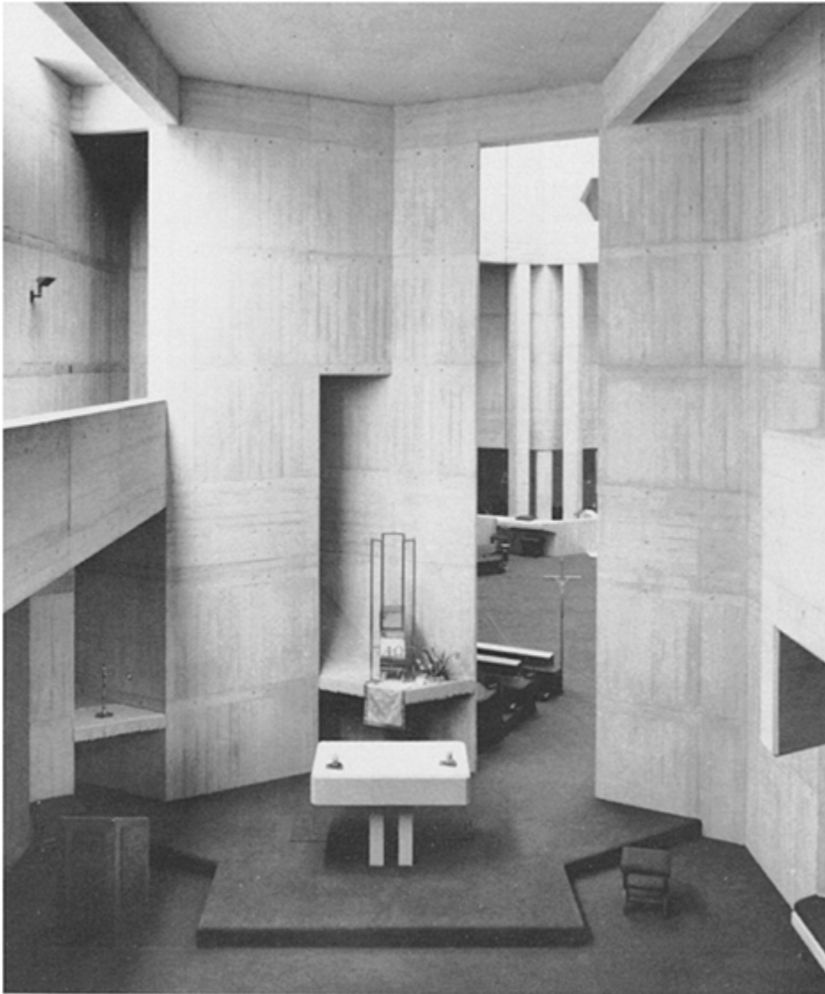
The skills of concrete placement and form design are evident in this board marked concrete work (J Laing Construction Company Limited)
