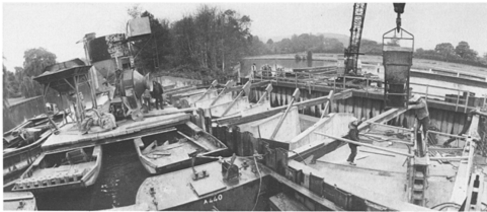
Taking the plant to the work—batching plant and mixer on barge adjacent to the point of placing
