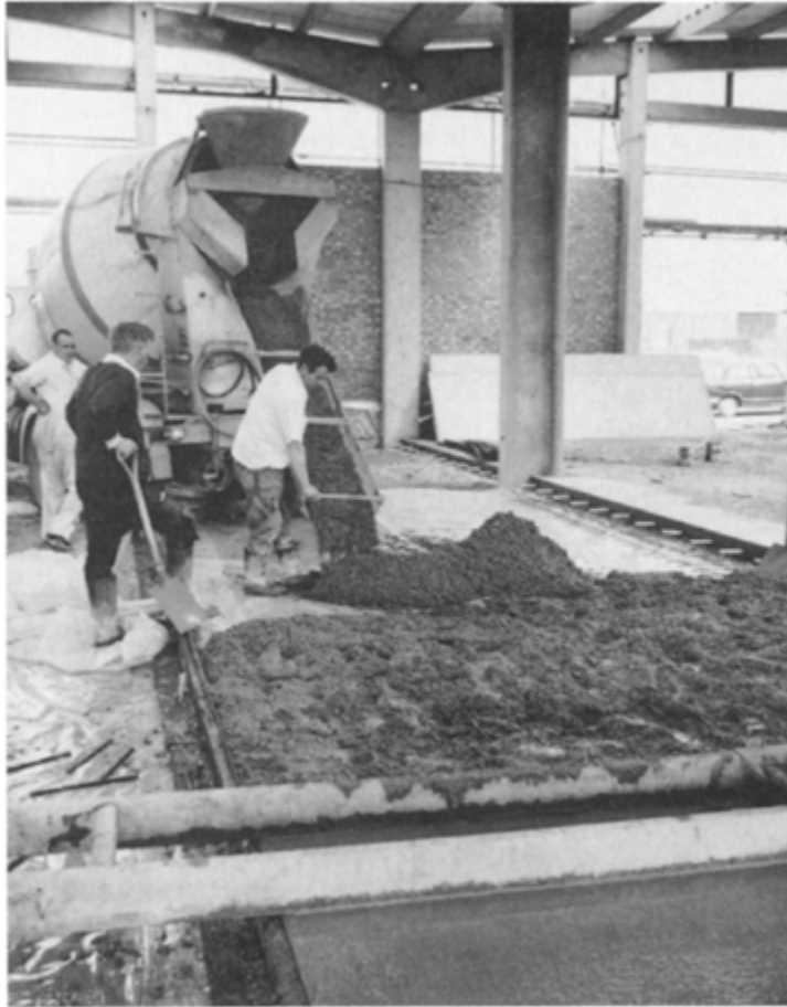
Readymixed concrete discharged at point of placement ready for screeding
