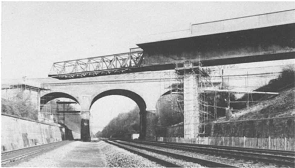
Bridge jacking—the launching process commences (British Railways)
