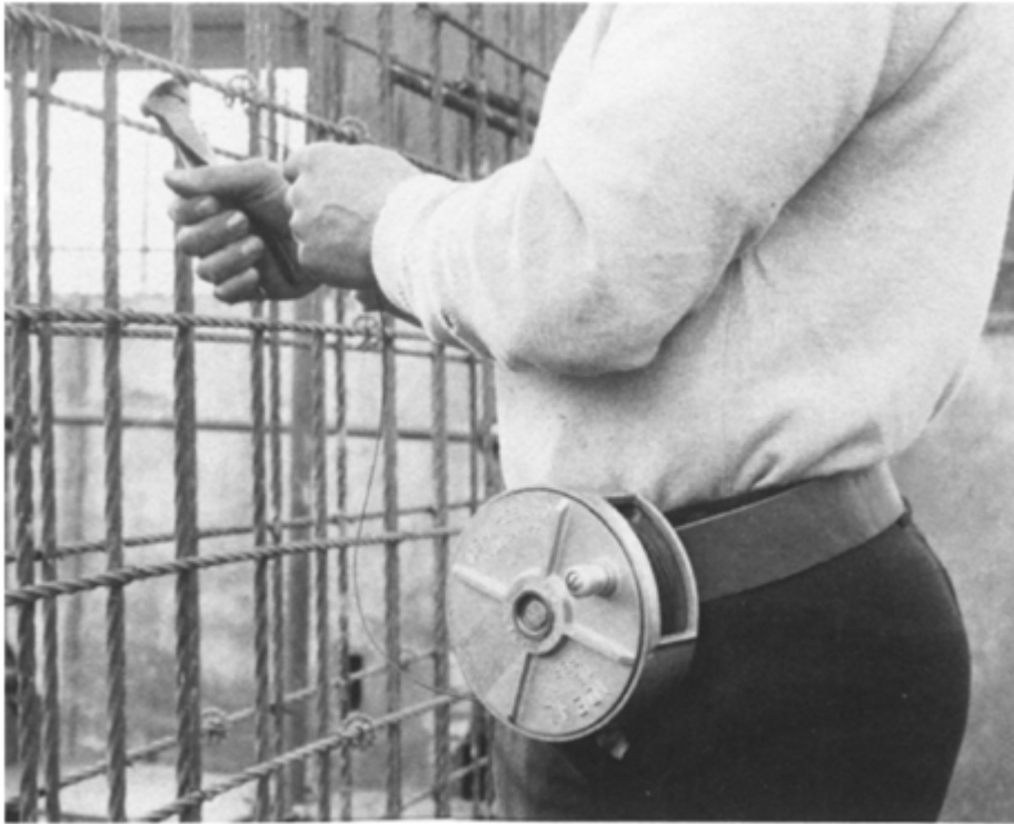
The ideal tie wire reel in use dispensing soft iron tying wire
