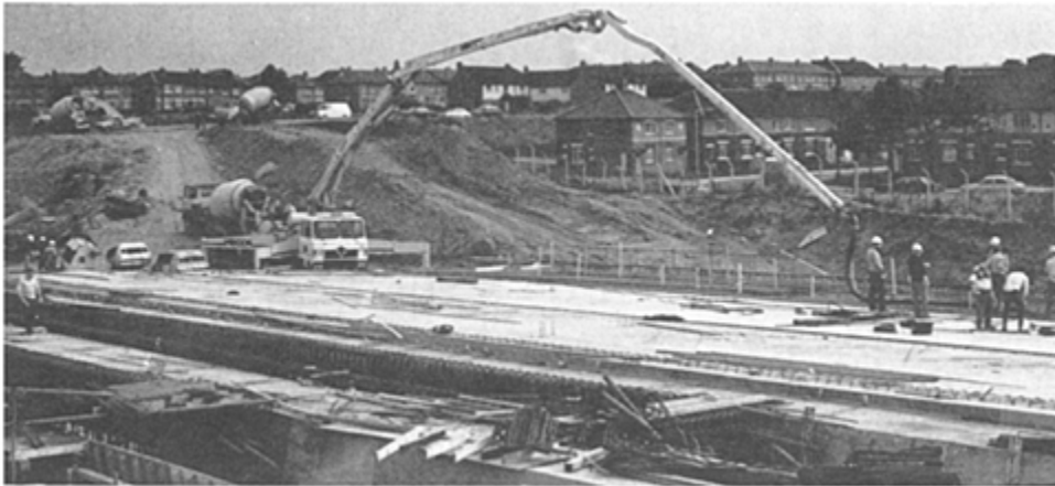
The ease of access achieved by the use of concrete pumping equipment is clearly shown in these illustrations of bridge construction—careful programming of delivery and adequate site preparation for readymixed concrete is essential (The Pochin Group)
