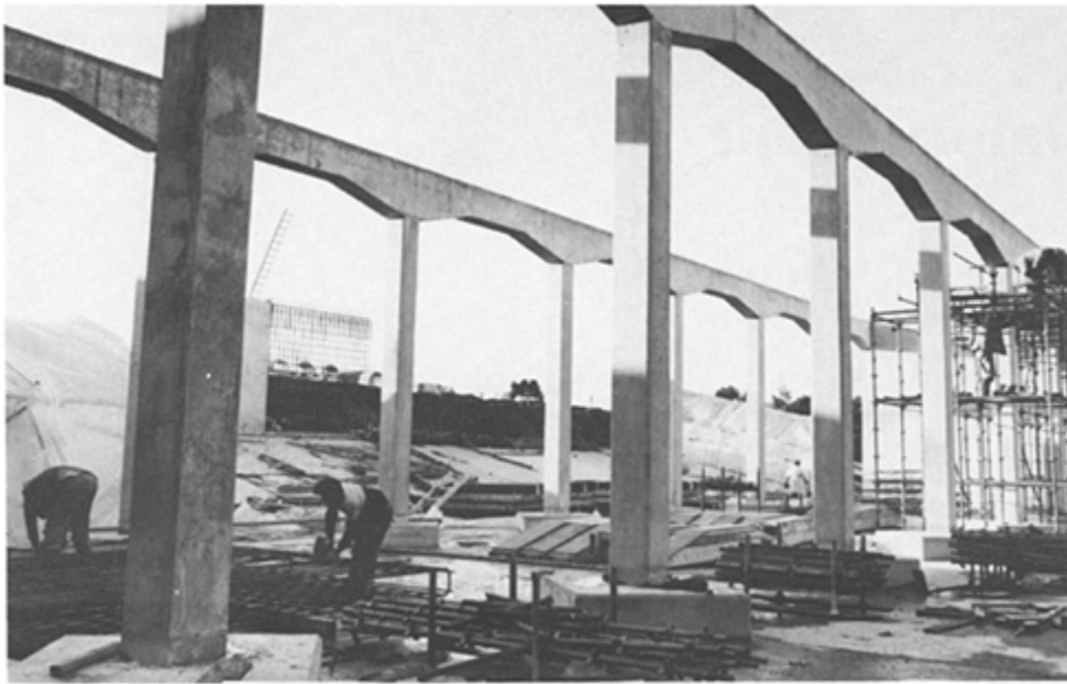
Steel fabrication for walls proceeding on a reservoir site (South West Water Authority)
