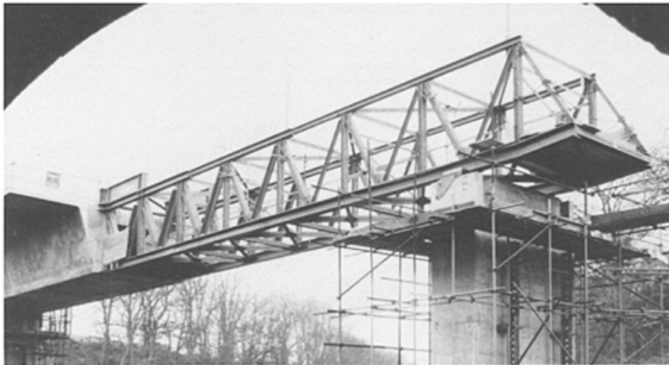
The launching nose—recoverable—reaches the first bridge pier (British Railways)
