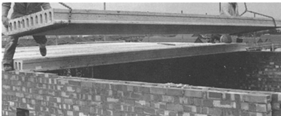
Prestressed concrete 'installation' wide slab units produced by machine on a long line bed (Bison Concrete Limited)
