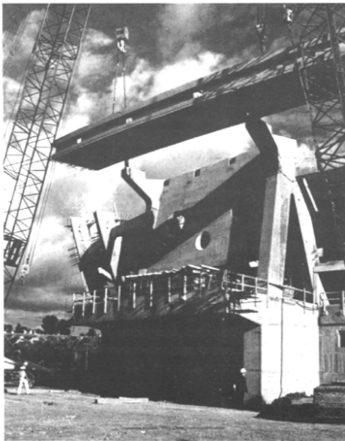
Erecting a pre-tensioned ring beam member (Jan Bobrowski and Partners)
