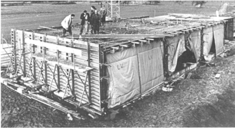
The tentage acts as container for free steam used in curing these system cast buildings (Uni-form Limited)
