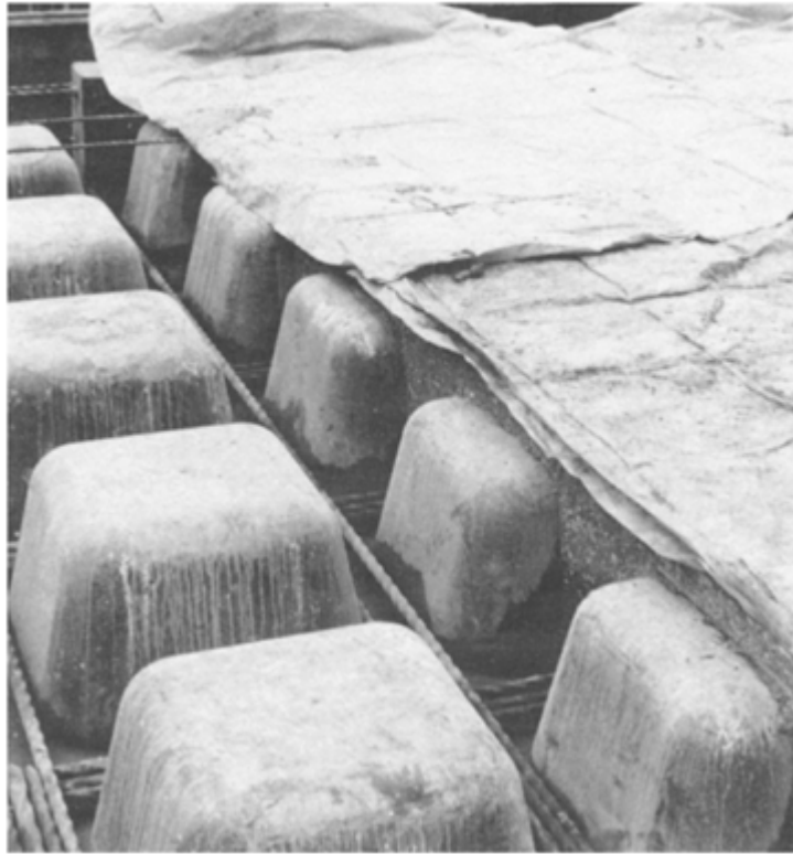
Curing waffle slab—note joint location and prepared joint face
