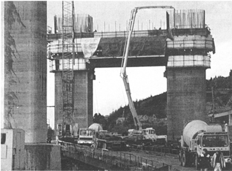
The ease of access achieved by the use of concrete pumping equipment is clearly shown in these illustrations of bridge construction—careful programming of delivery and adequate site preparation for readymixed concrete is essential (The Pochin Group)
