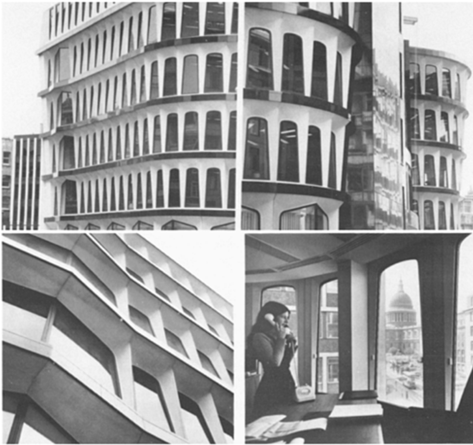
Glass reinforced cement is an emerging precast product as illustrated by these elements for a prestige office development (Wates Developments Limited)
