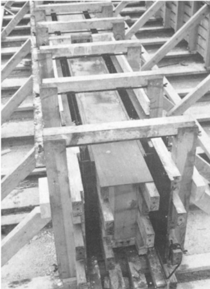
Precast mould of slender section prepared ready for filling
