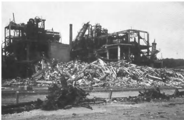
Figure 1.5. Damage to the Office Block and Process Areas at the Flixborough Works
