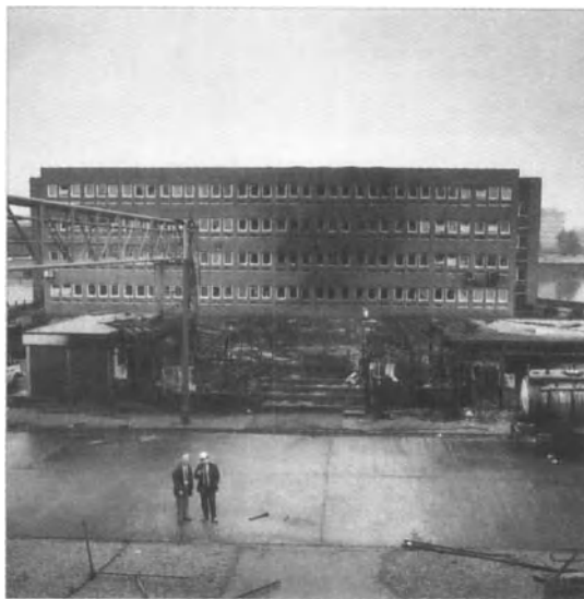
Figure 1.13. Damage to the Control Room and Impact on the Office Block from the Jet Flame at Hickson & Welch
