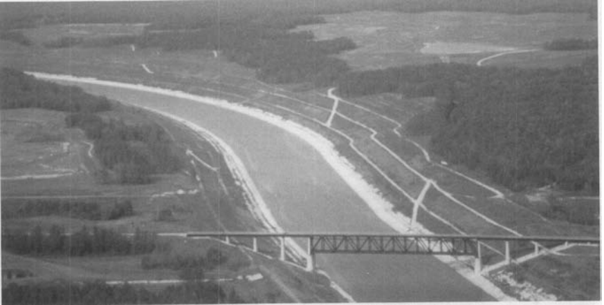
FIGURE 20-4. Tennessee-Tombigbee Waterway, Divide Cut.
