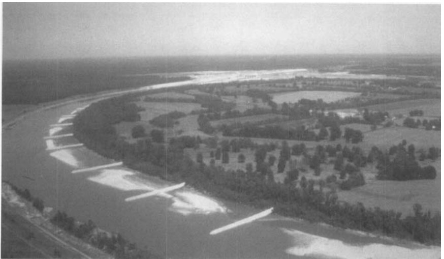
FIGURE 8-14. Stone Dike Field on Missouri River, 1987.
