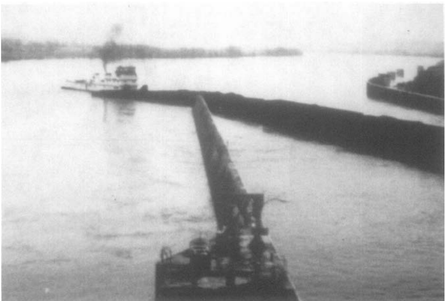
FIGURE 9-1. Tow Attempting to Enter Old Gallipolis Lock on Ohio River.
