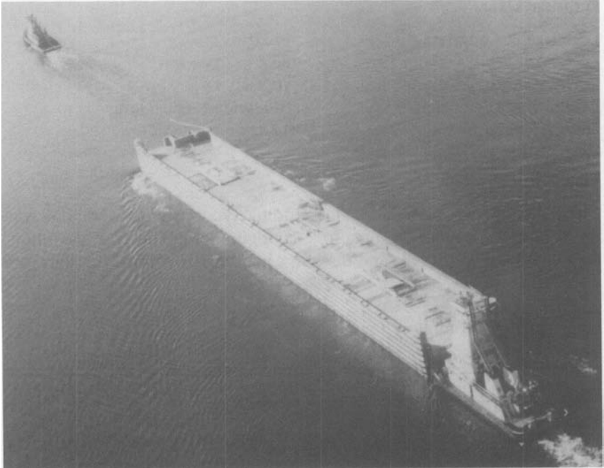
FIGURE 20-10. Bonneville Lock, 400 ft Long Floating Section of Upstream Guide Wall.
