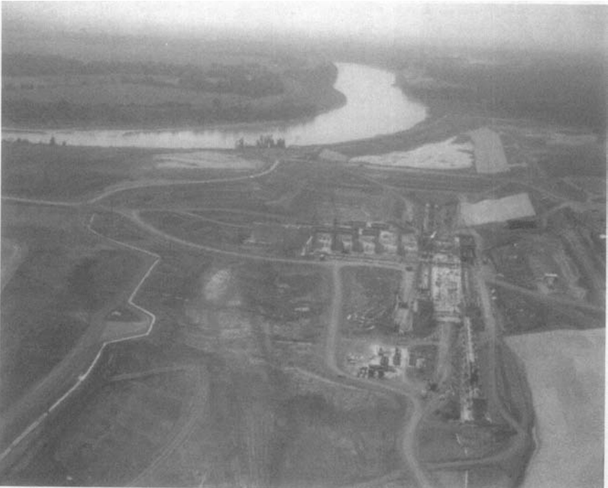
FIGURE 17-9. Red River Lock and Dam Construction in Bendway Cutoff.
