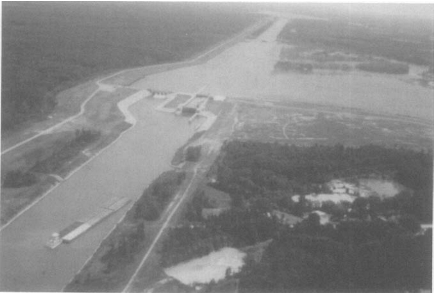
FIGURE 20-2. Tennessee-Tombigbee Waterway, Lock and Dam A: Canal Section.
