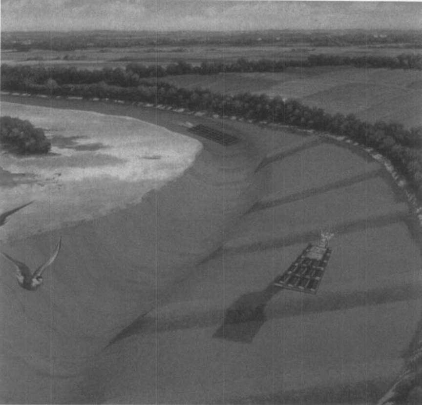
FIGURE 8-4. Bendway Weir.
