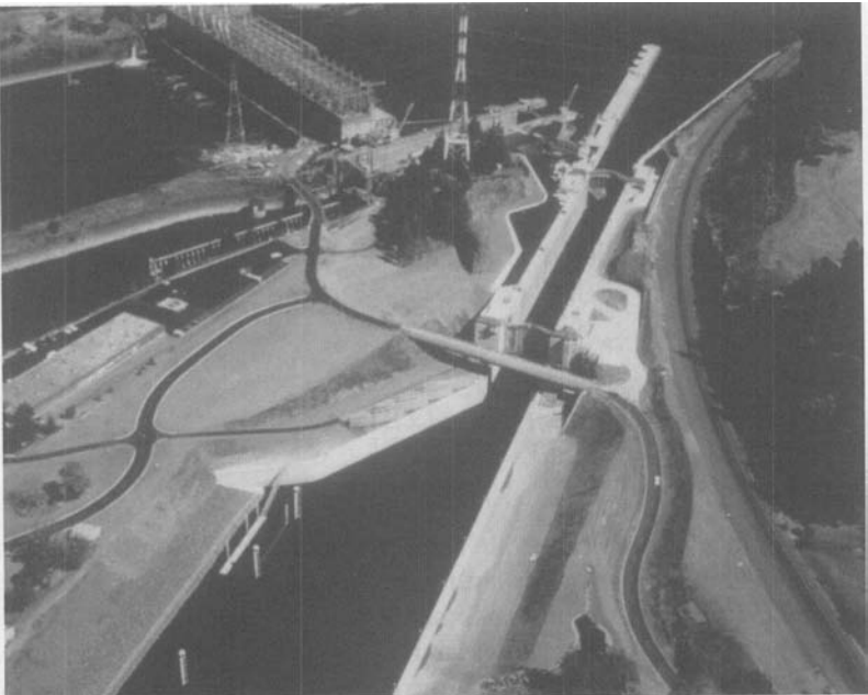
FIGURE 20-6. New Bonneville Lock.
