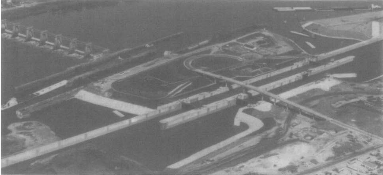
FIGURE 9-10. Robert C. Byrd Locks, Ohio River (Replacement for the Old Gallipolis Locks).
