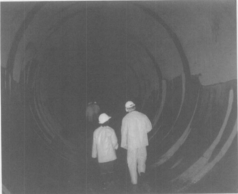
FIGURE 20-8. Bonneville Lock, Fill-and-Empty Conduits Mined Through Rock (15 ft dia).
