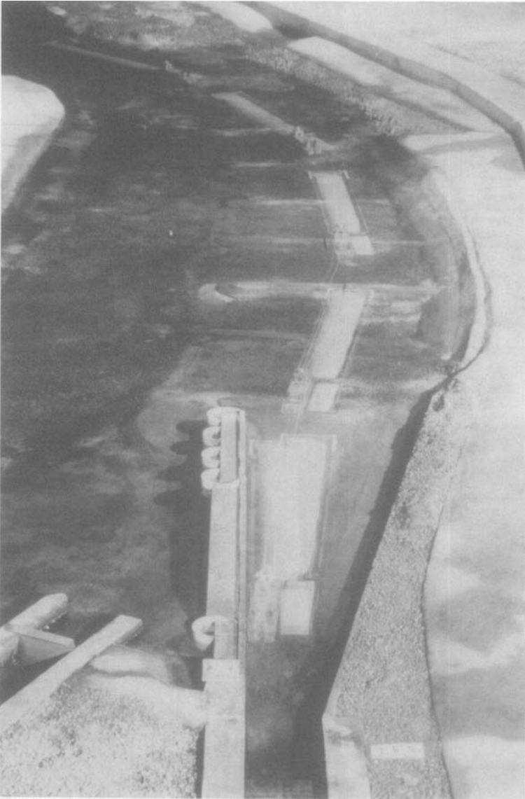
FIGURE 16-9. Upbound Tow Departing Bonneville Lock.
