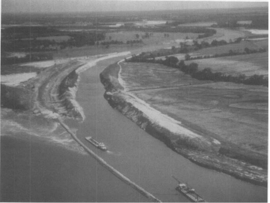
FIGURE 8-13. Channel Realignment on Red River, 1989.
