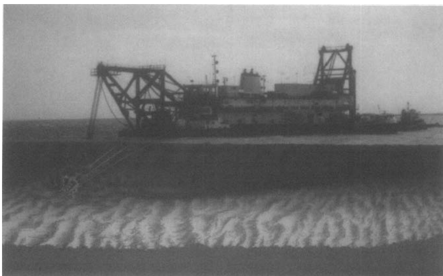
FIGURE 18-4. Cutterhead Pipeline Dredge with Underwater View.
