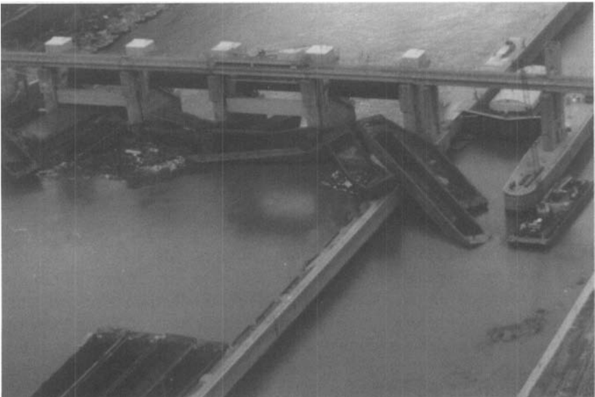
FIGURE 18-3. Accident at Maxwell Lock and Dam, Ohio River.
