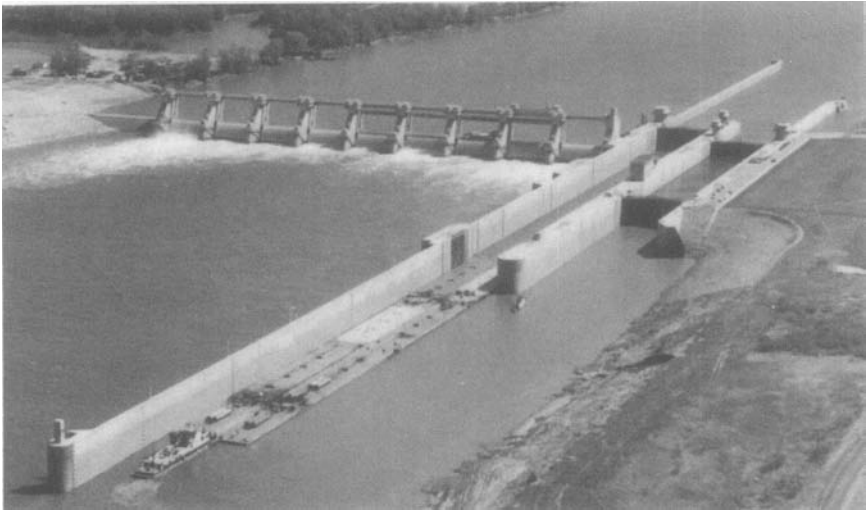
FIGURE 10-3. Parallel Locks with Gravity Walls. Willow Island Locks, Ohio River, with Design Lift of 20 ft.
