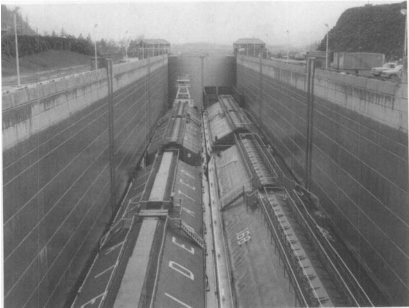
Figure 20-9. Bonneville Lock, Design Tow in Lock Chamber.
