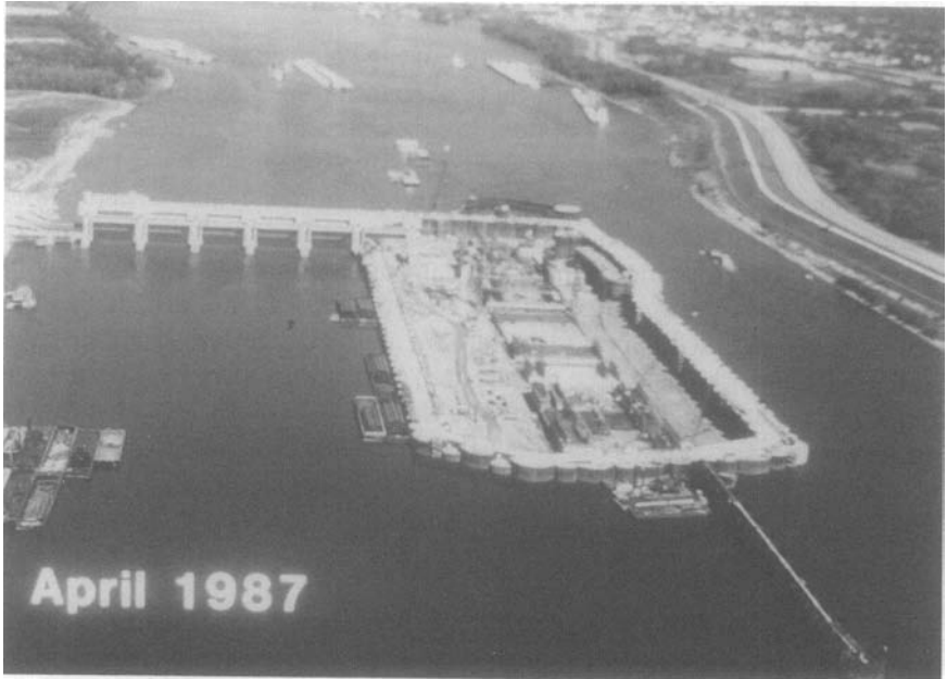
FIGURE 17-5. Second Phase, Melvin Price Lock and Dam.
