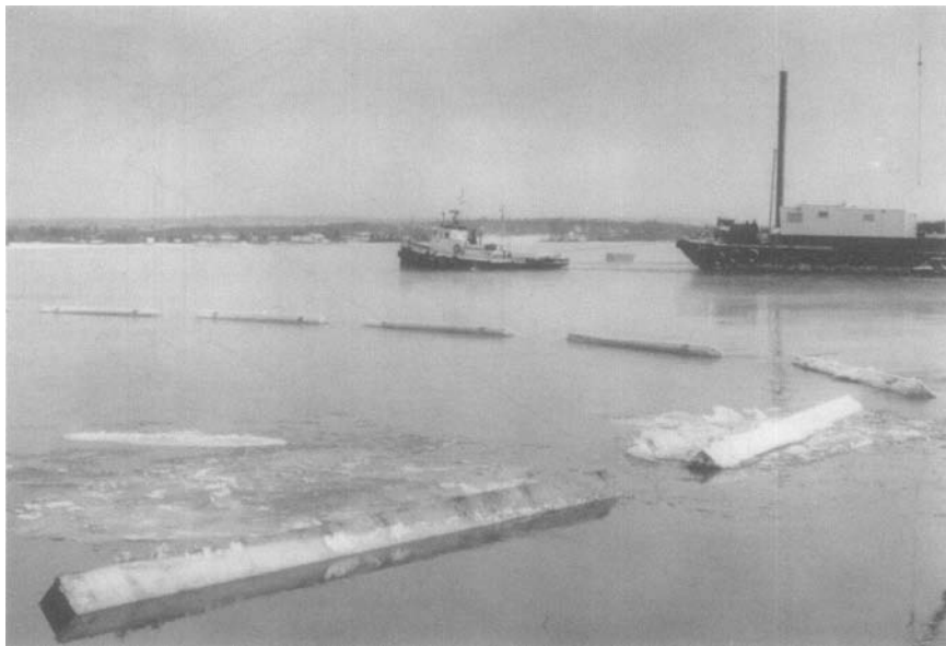
FIGURE 13-10. Timber Ice Boom.
