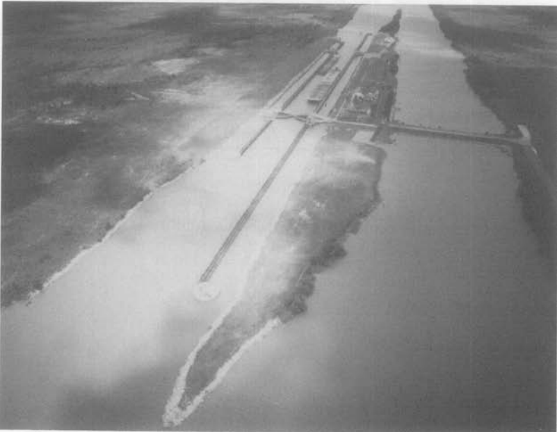
FIGURE 20-15. Leland Bowman Lock: (top) Lock Under Construction; (bottom) Completed Lock.
