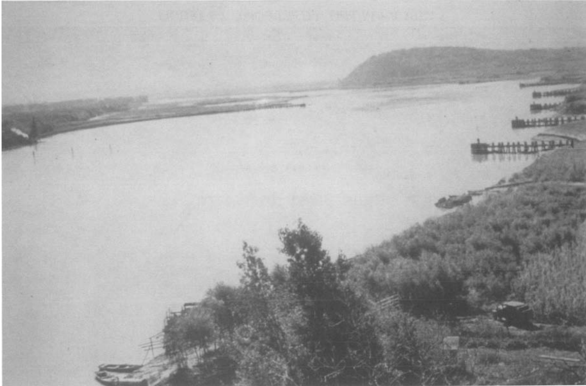
FIGURE 8-8. Dike Field Partly Filled, October, 1939.
