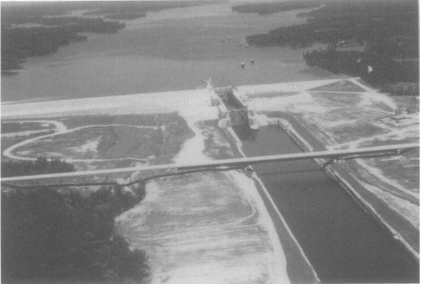
FIGURE 10-6. Lock with Thin Walls. Bay Springs Lock, Tennessee-Tombigbee Waterway, with Design Lift of 84 ft.
