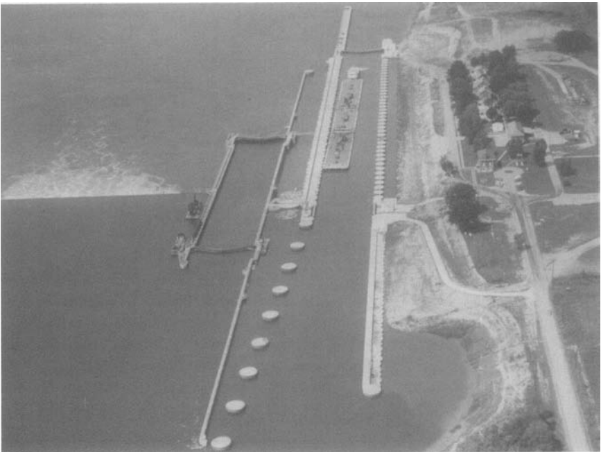
FIGURE 10-7. Temporary Lock with Cellular Sheetpile. Lock and Dam No. 52, Ohio River, with Design Lift of 12 ft.
