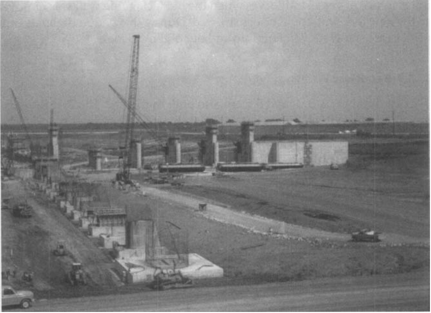
FIGURE 17-10. Red River Lock and Dam Construction in the Dry.
