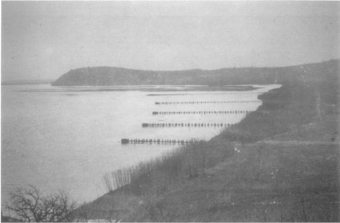
FIGURE 8-7. Timber Pile Dike Field, March, 1935.
