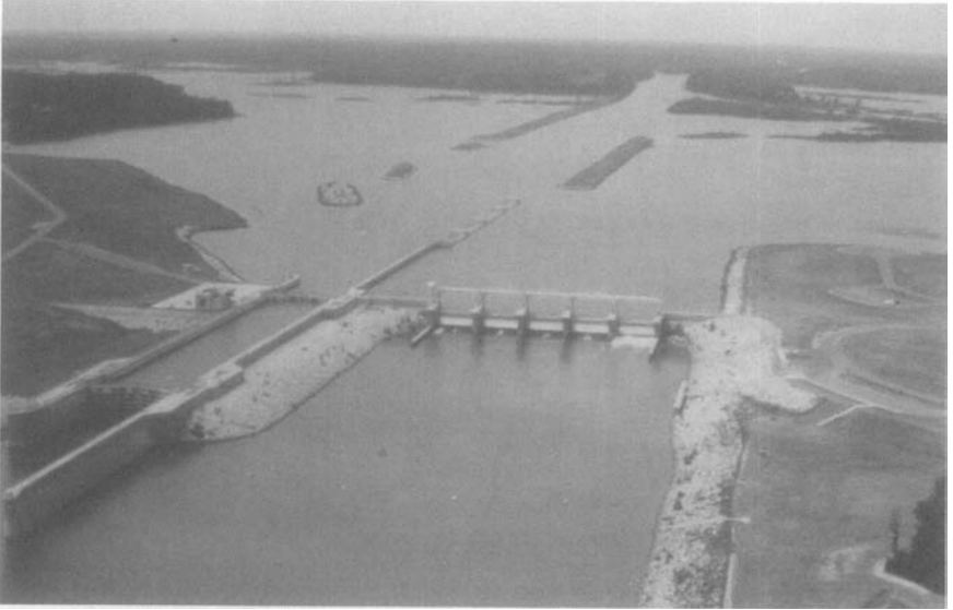
FIGURE 20-1. Tennessee-Tombigbee Waterway, Columbus Lock and Dam: River Section.
