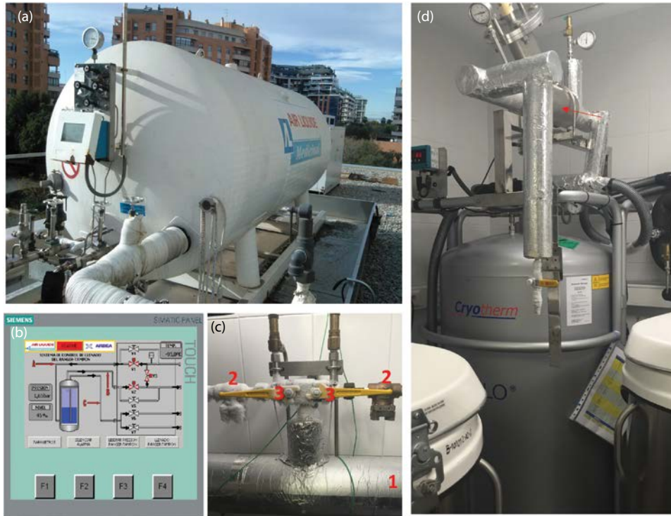
Figure 24.4 (a) Reservoir tank for liquid nitrogen (LN) storage (Air Liquide, Madrid, Spain). (b) Detail of the touchscreen controller of the system, showing the scheme for the filling of the pressurized tank. The filling of the pressurized tank (Apollo 350, Cryotherm, Kirchen (Sieg), Germany) begins at -130^{\circ}\text{C} and is controlled by the system by actuating three solenoids (V1, V2, and V3). All the LN-phase gas coming from the reservoir tank via pipe A is disposed of in order to ensure that the pressurized tank is filled with liquid-phase nitrogen. The LN fills the pressurized tank (nurse tank) when the preset temperature is reached. The excess pressure generated during the filling phase is removed via pipe B. The valves automatically close when the filling is completed. LN is supplied to the vapor storage tanks via specific pipe C. In case of failure, the system can be handled manually by the action of the manual solenoids V4, V5, V6, and V7. (c) (1) Pipe with insulating coating for LN; (2) online wire mesh pre-filter; (3) entry valve for each tank. (d) Pressurized (nurse) tank. The arrow shows the ceramic filter Ceralin online.
