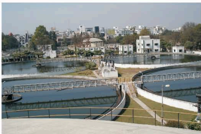
Secondary Sedimentation Tank
