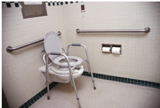
FIG. 18-7 Handrails and an elevated toilet seat make transfers easier for the patient.
