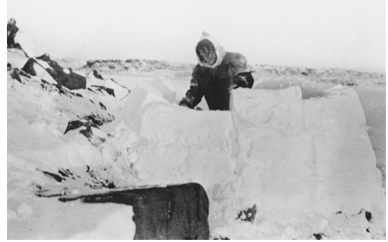
A small igloo that was used as a temporary shelter by hunters could be built by one person in about two hours. (Canadian Geological Survey/Library of Congress, Prints and Photographs Division [LC-USZ62-103522])
