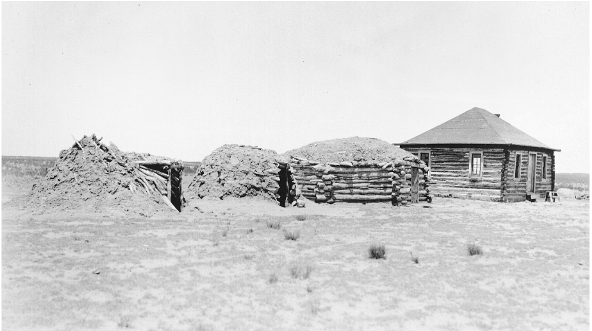
Early hogans were covered with earth, which served as an insulator against heat and cold. Later the Navajo (Dineh) people began building the sides out of logs and covering only the roof with earth. The house in the background was considered a modern hogan when this picture was taken in 1938 at the Southern Navajo Agency. (National Archives and Records Administration Pacific Alaska Region/Photograph No. NRIS-75-PAO50-NAVHOME4)
