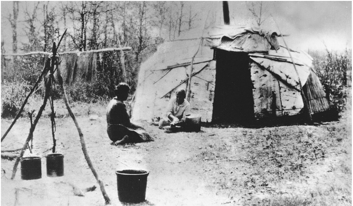
Women from the Consolidated Chippewa Agency in Minnesota sit in front of a dome-shaped wigwam. It is covered with sheets of birch bark. On the right it is covered with a woven mat of rushes or cattails. This picture was taken in 1915. (National Archives and Records Administration Central Plains Region/Photograph No. NRE-75-COCH[PHO]-623)
