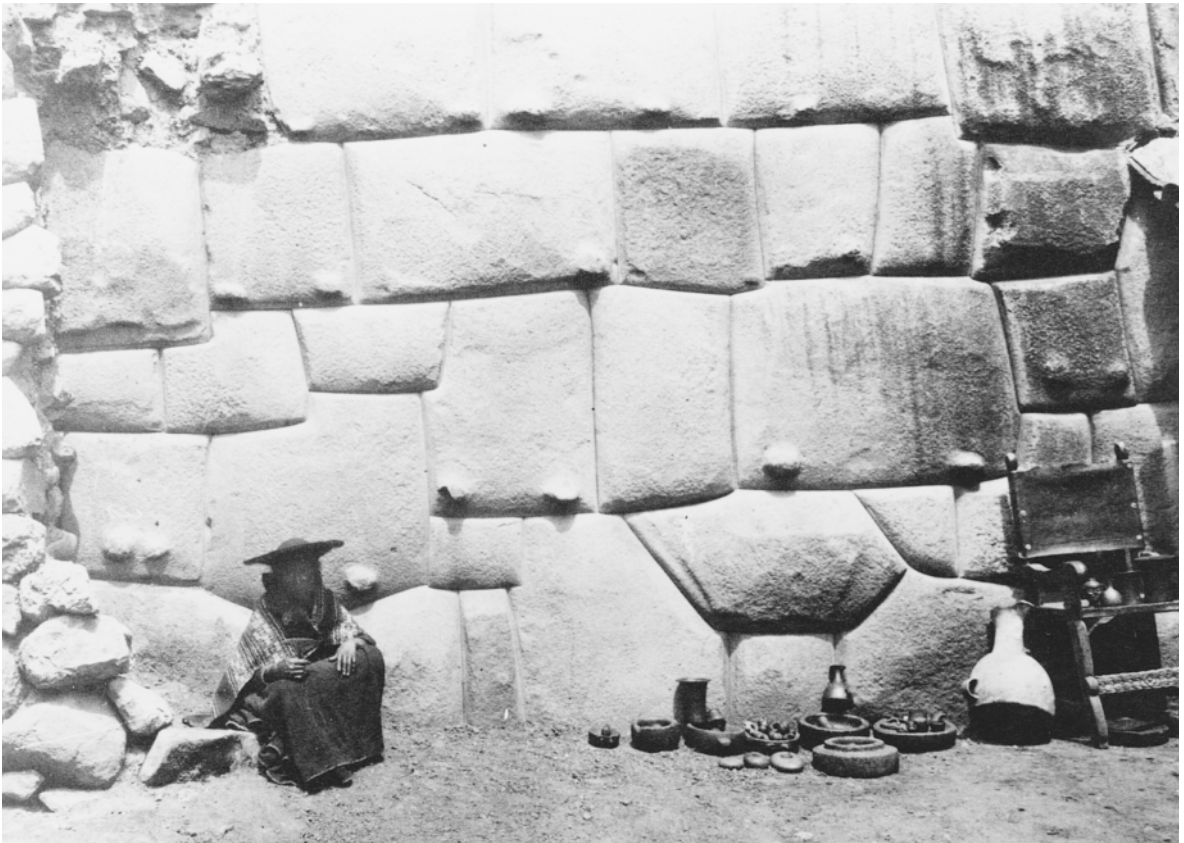
Inca stonemasons carved stones and set them carefully. They were such skilled builders that after hundreds of years it is still impossible to push a razor blade between the stones. ( Library of Congress, Prints and Photographs Division [LC-USZ62-97754] )
