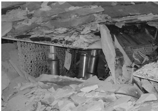
Figure 22-1 Mining tunnel cave-in. Underground mining has one of the highest fatal injury rates of any U.S. industry—more than five times the national average compared with other industries. Between 1999 and 2008, almost 40% of all underground fatalities were attributed to mine roof, rib, and face falls. (From http://www.cdc.gov/niosh/mining/topics/images/rockfall.jpg .)
