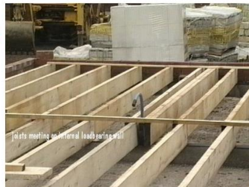
Construction of Suspended timber floors
