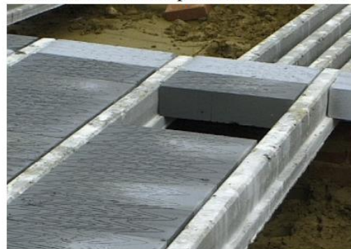
Suspended concrete beam and blocks
