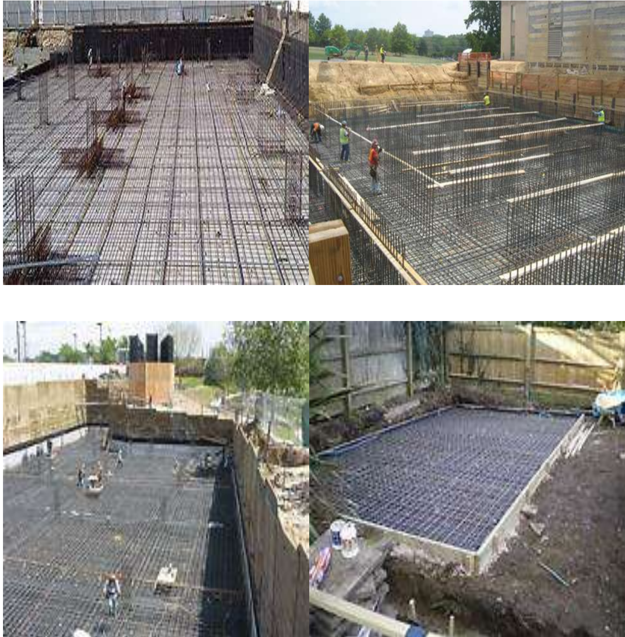
Figure: Typical View of Mat Foundation
