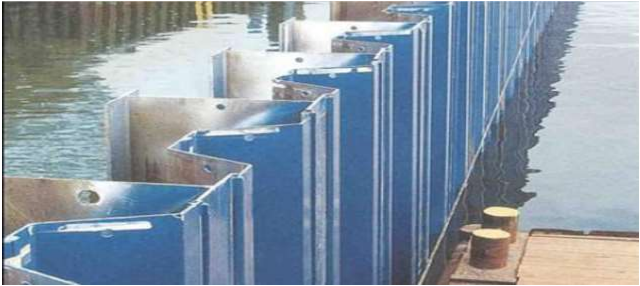
Figure 5.17 Sheet pile Walls
