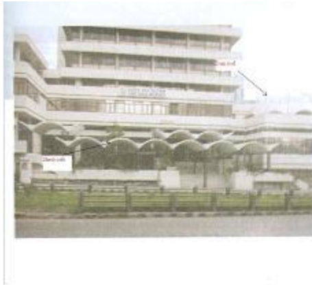
Fig. Shell and Domeroofs of EIC office building in A.A.
