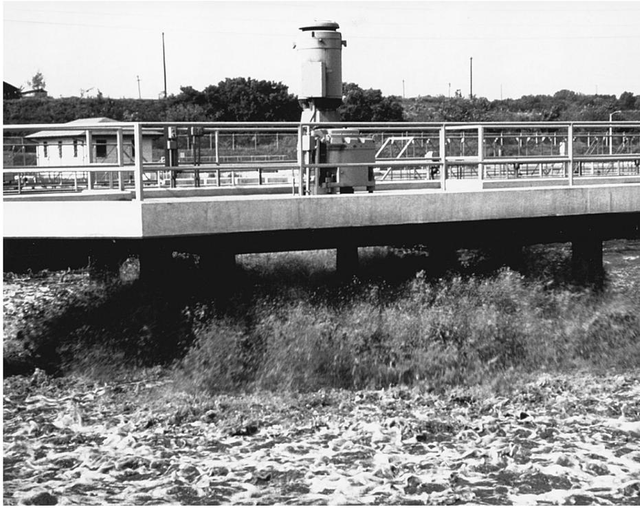
FIGURE 38 Platform-mounted low-speed mechanical aerator with an inverted open cone for high oxygen-transfer efficiency in an extended-aeration activated-sludge process. Source: EIMCO Process Equipment.
