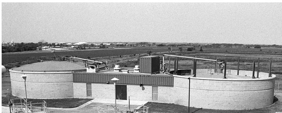
FIGURE 13 Sketch of a two-stage anaerobic digestion system. (a) The first stage is a completely mixed high-rate digester with a fixed cover. The second stage is a thickening and storage tank covered with a dome for collecting and storing gas. (b) Photograph of two-stage digesters, Lincoln, NE.
