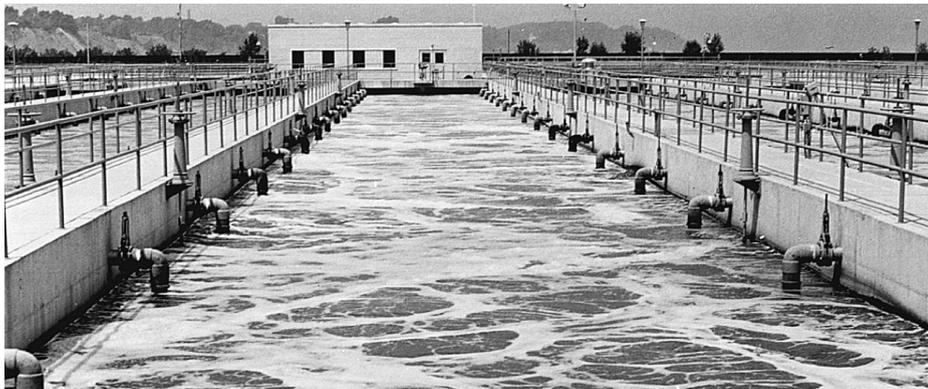
FIGURE 34 Fine-bubble diffuser for wastewater aeration. (a) A disc diffuser mounted on top of an air distributor pipe. (b) A grid of diffusers attached to air pipes mounted on the floor of an aeration tank. (c) Long rectangular aeration tank with uniform mixing and oxygenation by a grid of fine-bubble diffusers. *Source:* Sanitaire, a division of ITT Industries, Inc.
