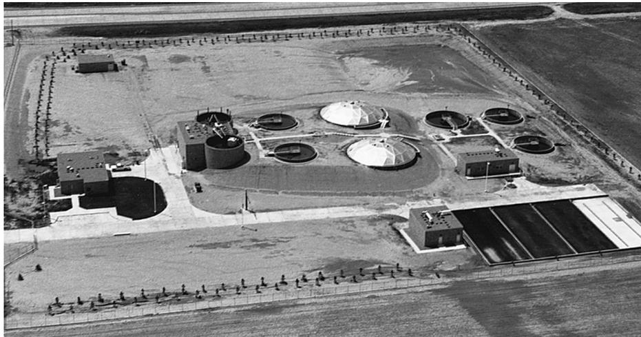
FIGURE 6 Aerial view of two-stage filter plant shown in Figure 5. Note domes on trickling filters to prevent ice formation. *Source:* HDR Engineering, Inc.
