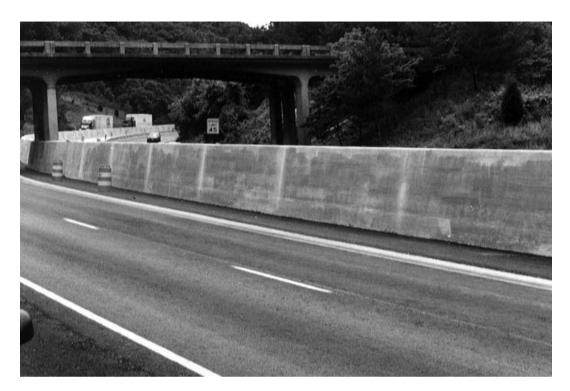
Figure 15.7 Single-Slope Concrete Median Barrier
