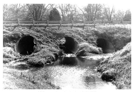
(a) Corrugated metal arch culvert (ARMCO)
