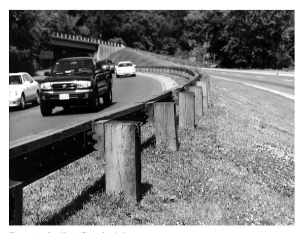
Figure 15.6 Steel-Backed Timber Guardrail
