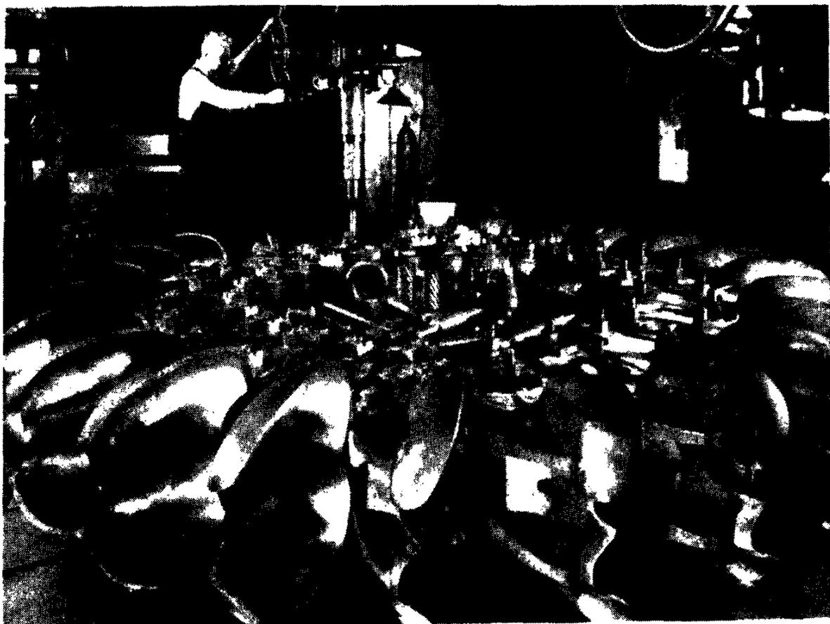
FIG. 8.11. Southern California Edison, Big Creek 2A, 1948.  $8\frac{1}{2}$ -in.-diameter jet impulse buckets and disk in process of being reamed. 56,000 hp, 2200 ft head, 300 rpm. (*Allis-Chalmers Mfg. Co.*)
