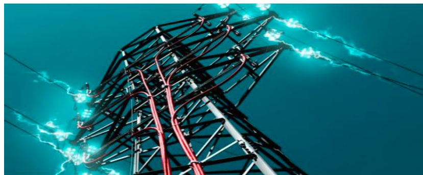
Figure 1.2 Electricity transmission line
