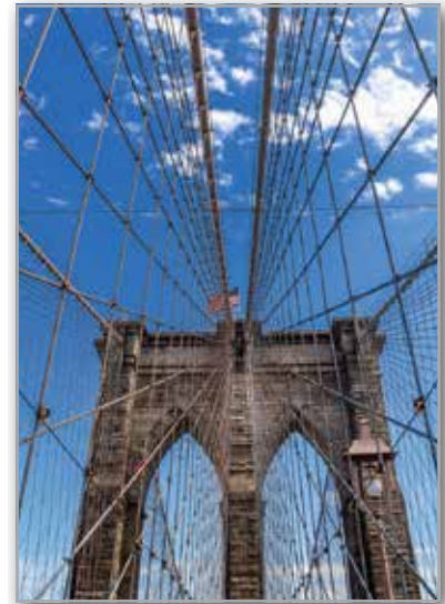
Breaking Strength (Exercise 102, p. 360)
