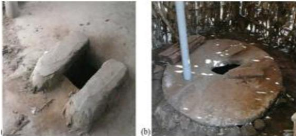
Figure 7.2: (a) Slab with raised footrest in a pit latrine. (b) Round cement slab
