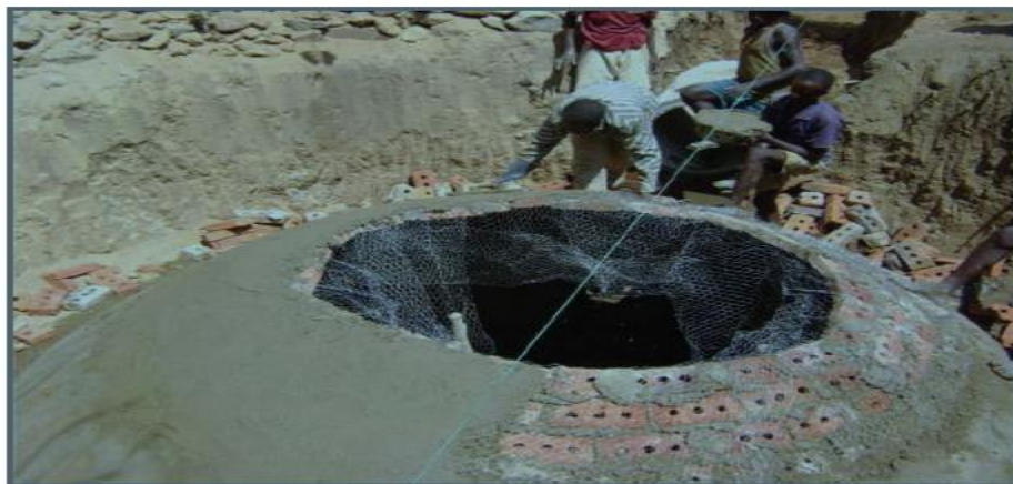
Figure 19.6:- An anaerobic digester under construction
