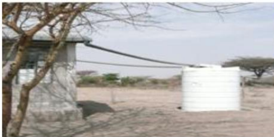
Figure 9.1:- Rainwater is collected from the roof of this health centre and stored in a covered, Water tight.
