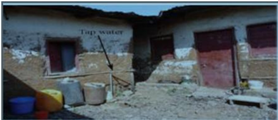
Figure 6.3:- Provision of safe water for a household with a single tap – an example of intermediate access.
