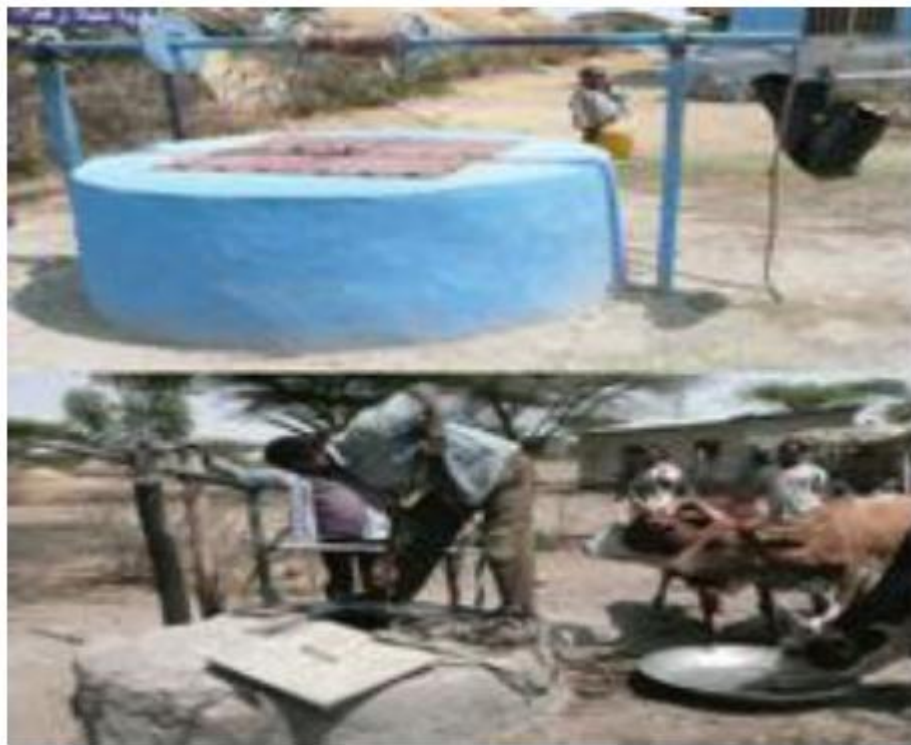
Figure 7.5: Two wells with concrete protection.
