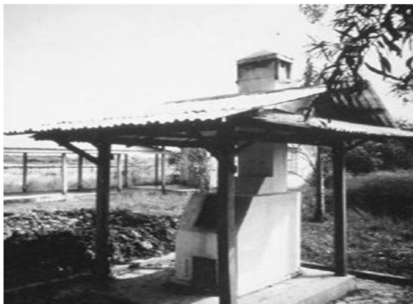
Figure 5.2: Single-chamber incinerator (on the left) and drum incinerator with chimney (on the right)
