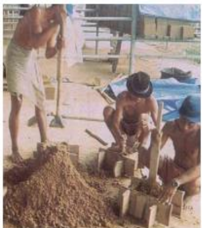
Molding using wooden bars
