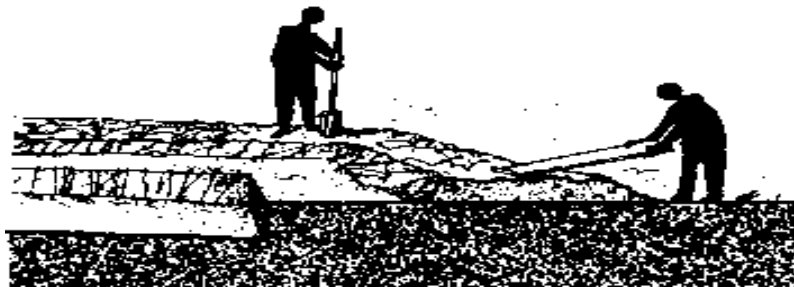
Fig .6 Compacting the pond dyke(embankment)
