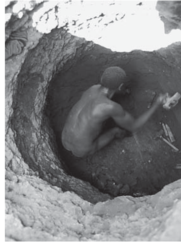
Fig. 13. Digging a well with hammers and iron sticks.
