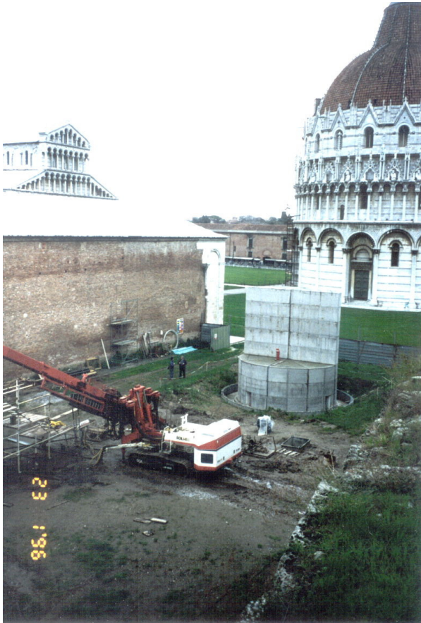
Figure 15 Underexcavation trial field
