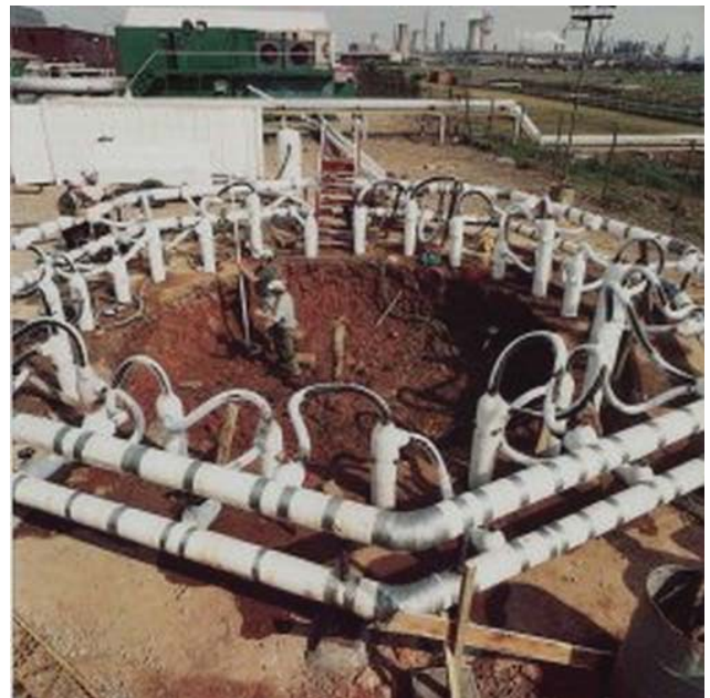
Figure 26.11 Ground freezing. (Courtesy of British Drilling and Freezing Co. Ltd.)
