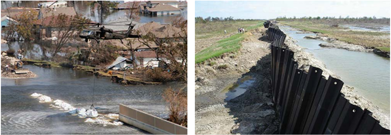
Figure 1.9 New Orleans levee failures during the Katrina hurricane in 2005. (Courtesy of United States Army Corps of Engineers.)
