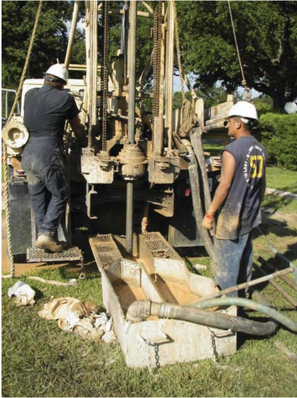
Figure 6.3 Wet rotary drilling method including mud pit. (Right: Courtesy of Wikimedia. See also this video: http://cee.engr.ucdavis.edu/faculty/boulanger/video.html )
