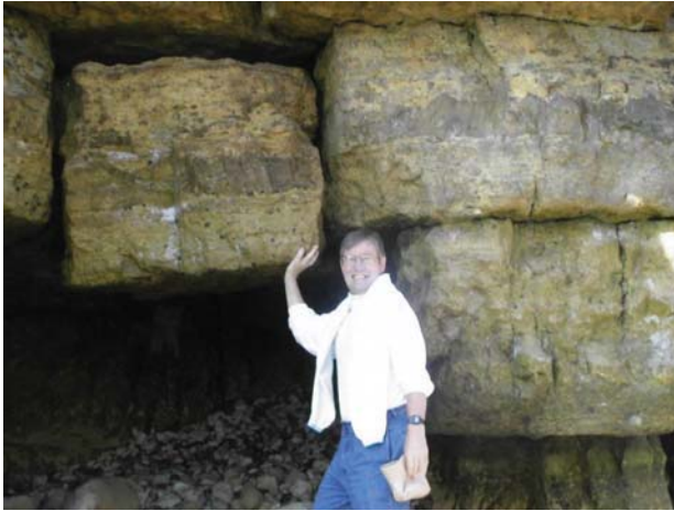
Figure 5.12 Jointed rock mass and caverns at Pointe du Hoc.
