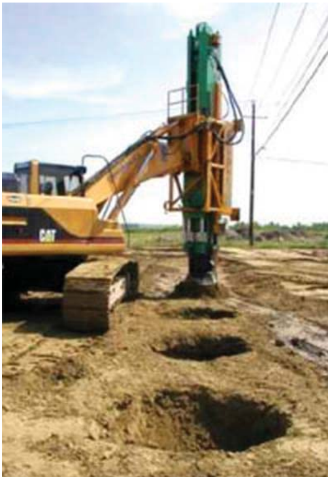
Figure 26.3 Example of rapid impact compactor. (Courtesy of Menard Bachy, Inc.)
