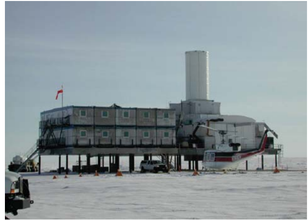
Figure 5.16 Elevated structure on permafrost. (Courtesy of Anadarko Petroleum Corporation.)
