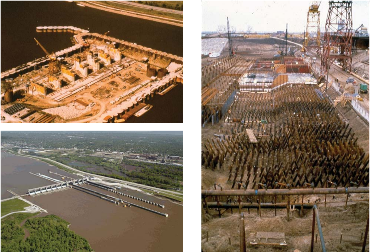
Figure 1.5 Lock and Dam 26 on the Mississippi River in 1990. (a: Courtesy of United States Army Corps of Engineers, b: Courtesy of Thomas F. Wolff, St. Louis District Corps of Engineers, 1981. c: Courtesy of Missouri Department of Transportation.)
