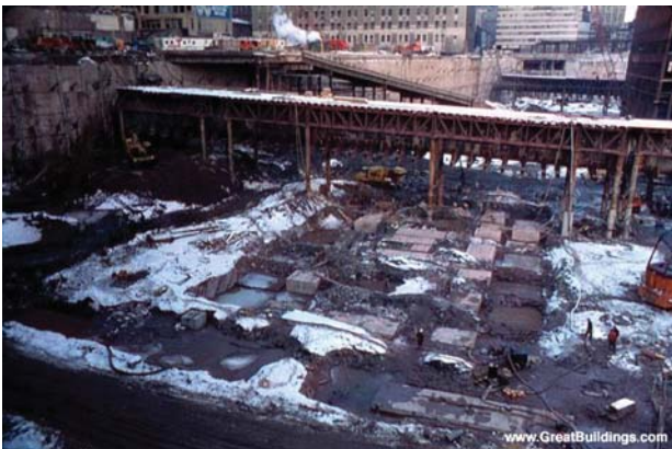
Figure 5.10 Photo of the foundation for the World Trade Center. (Courtesy of the Port Authority of New York and New Jersey.)
