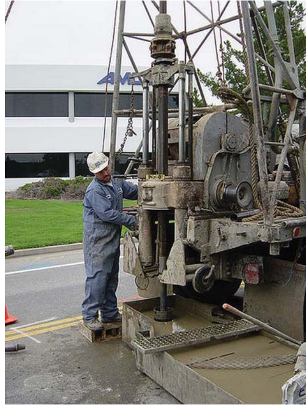
Figure 6.3 Wet rotary drilling method including mud pit. (Right: Courtesy of Wikimedia. See also this video: http://cee.engr.ucdavis.edu/faculty/boulanger/video.html )
