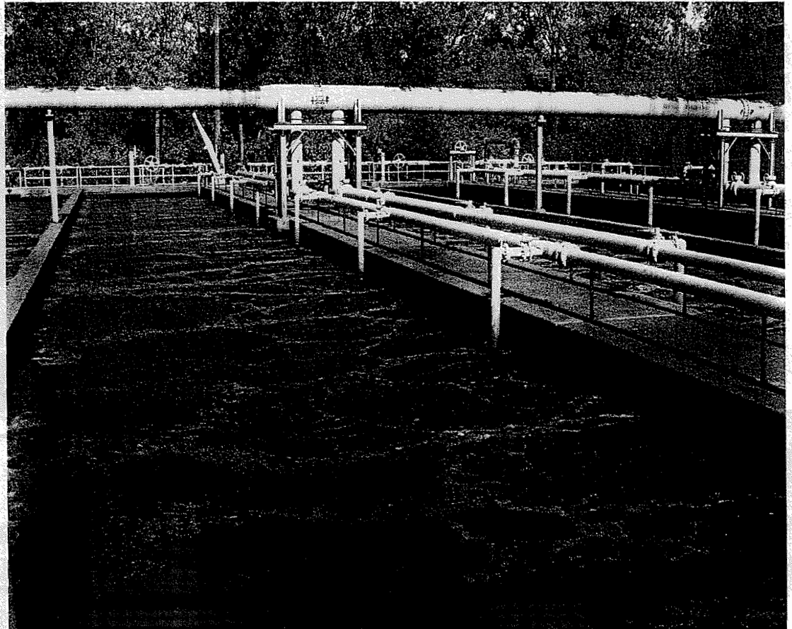
FIGURE 6-20 Activated sludge aeration tank under air. (Source: E. Lansing WWTP, photo courtesy of Harley Seeley of the Instructional Media Center, Michigan State University.)
