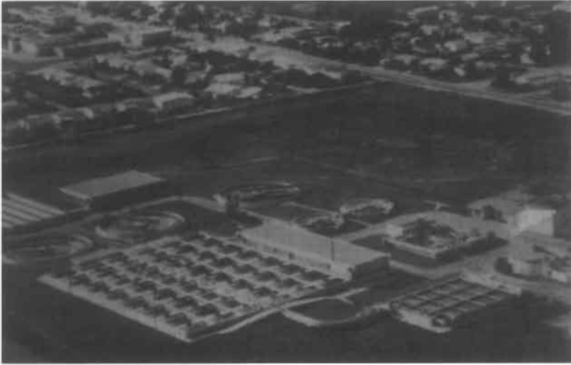
Figure 9-22. An aerial view of a secondary wastewater treatment plant. (Courtesy of Envirex.)
