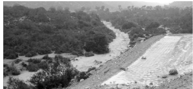
Figure 29.10 Ephemeral drainage channel in flood after a storm; note the proximity of the drainage channel to the newly placed earthwork places the earthwork at risk Reproduced from Truslove (2010); all rights reserved
