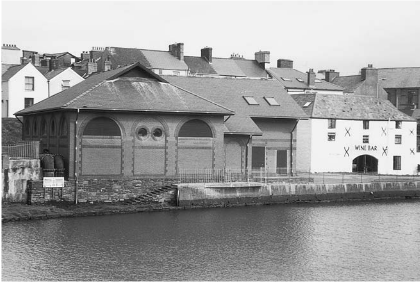
Fig. 14.11 Pumping station: architectural treatment
