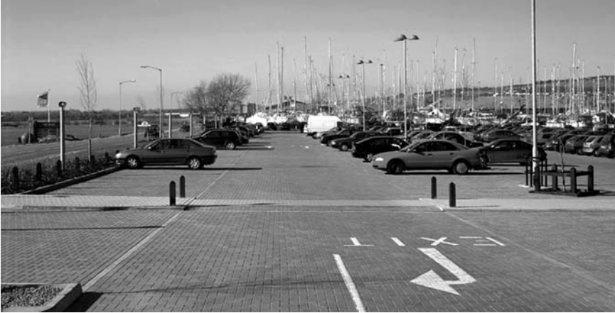
Fig. 21.5 Car park with pervious pavement (courtesy of Formpave Limited)
