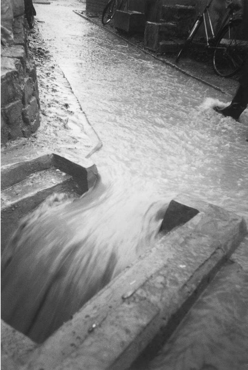
Fig. 23.7 Road-as-drain in Indore, India
