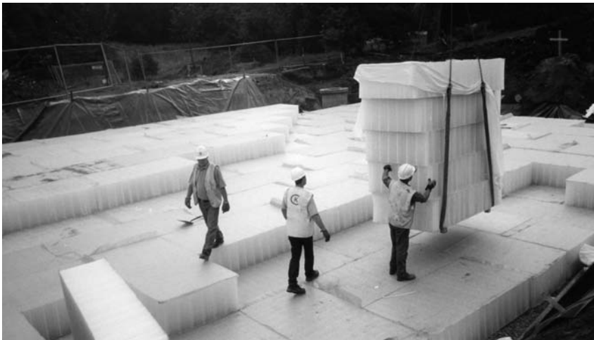
Fig. 13.2 Installation of a Stormcell® storage device (courtesy of Hydro International)
