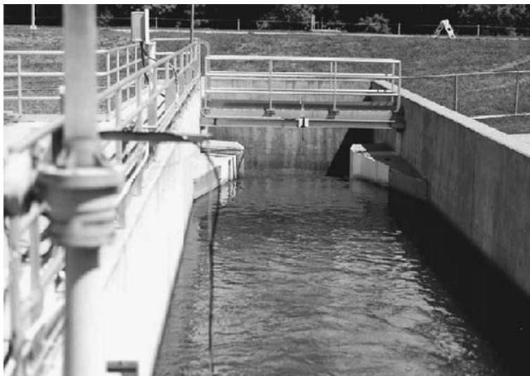
Fig. 4.18 – Chlorine contact tank (courtesy of Sydney Water, Australia)
