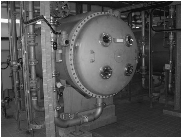
Fig. 4.15 – Ozone generator (courtesy of Anglian Water, UK)
