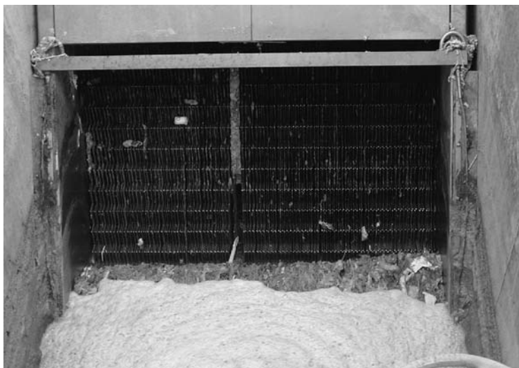
Fig. 3.15 – Screening of raw sewage (courtesy of Anglian Water, UK)
