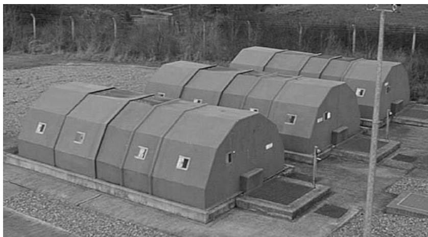
Fig. 6.7 – Rotating biological contactor (courtesy of Severn Trent Water, UK)
