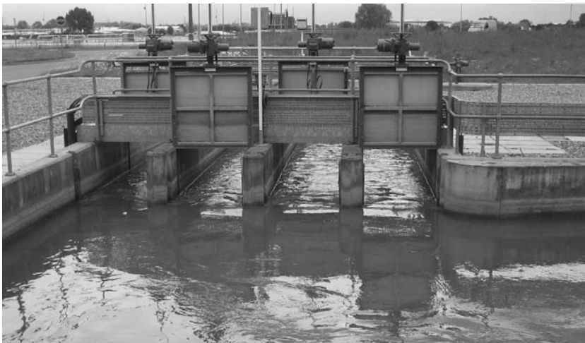
Fig. 3.4 – Constant velocity channels (courtesy of Anglian Water, UK)
