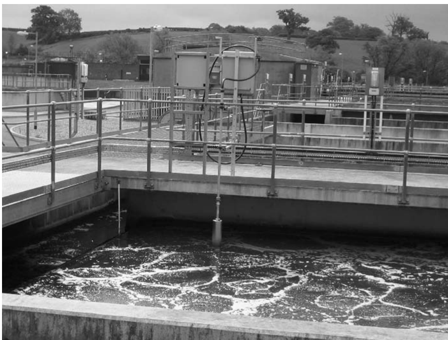
Fig. 1.4 – In-situ ammonia monitoring of an activated sludge aeration lane (courtesy of Severn Trent Water, UK)
