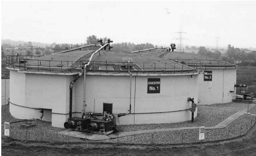
Fig. 8.5 – Sludge digesters (courtesy of Anglian Water, UK)
