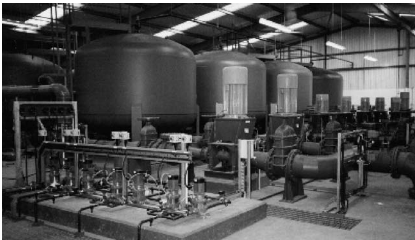
Fig. 3.27 – Battery of pressure filters (courtesy of Anglian Water, UK)
