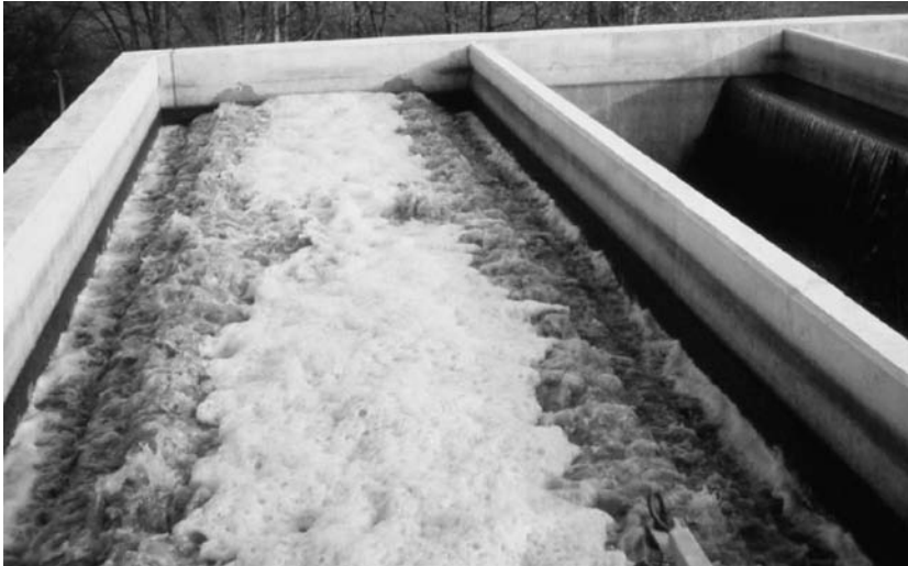
Fig. 3.26 – Air scouring of a rapid gravity filter (courtesy of Thames Water, UK)
