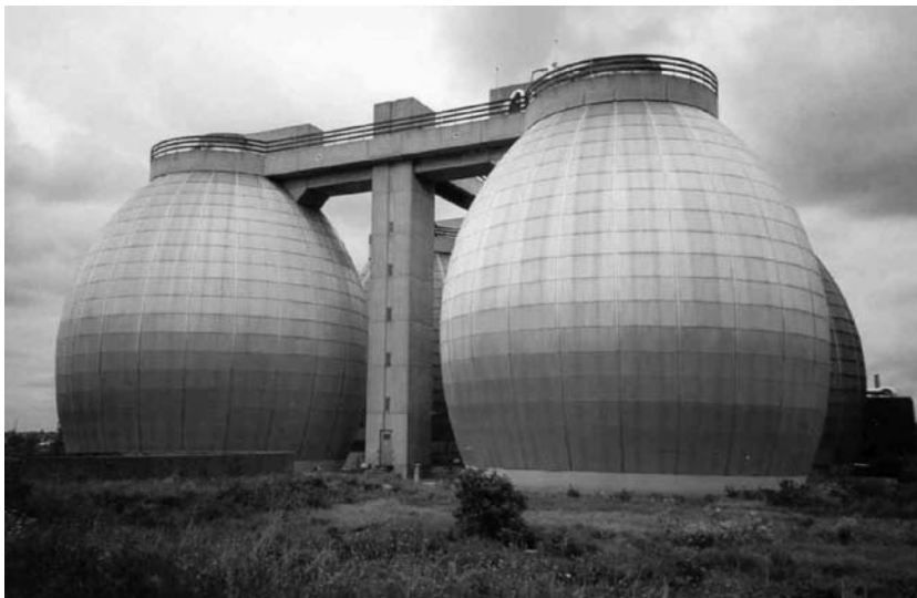
Fig. 8.9 – Egg-shaped anaerobic digester (courtesy of Avedoere Wastewater Services, Denmark)
