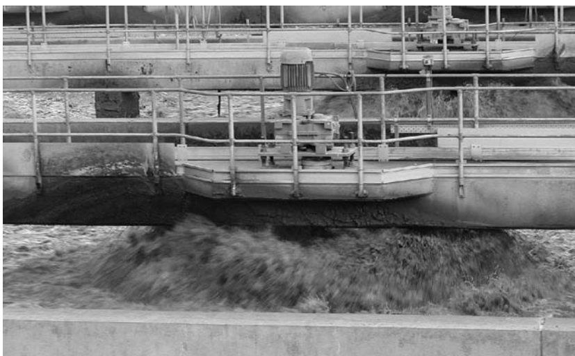
Fig. 6.11 – Activated sludge surface aeration (courtesy of Anglian Water, UK)
