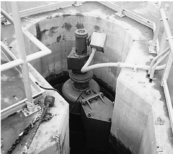
Fig. 3.22 – Comminutor (courtesy of Yeomans Chicago Corporation, USA)
