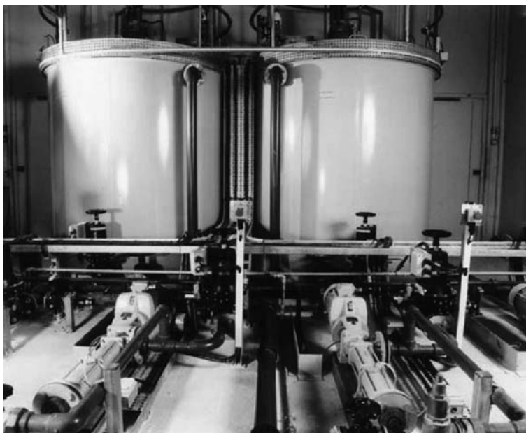
Fig. 4.1 – Dosing pumps and storage tanks (courtesy of Anglian Water, UK)
