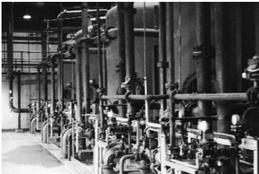
Fig. 5.5 – Industrial two-bed deioniser
