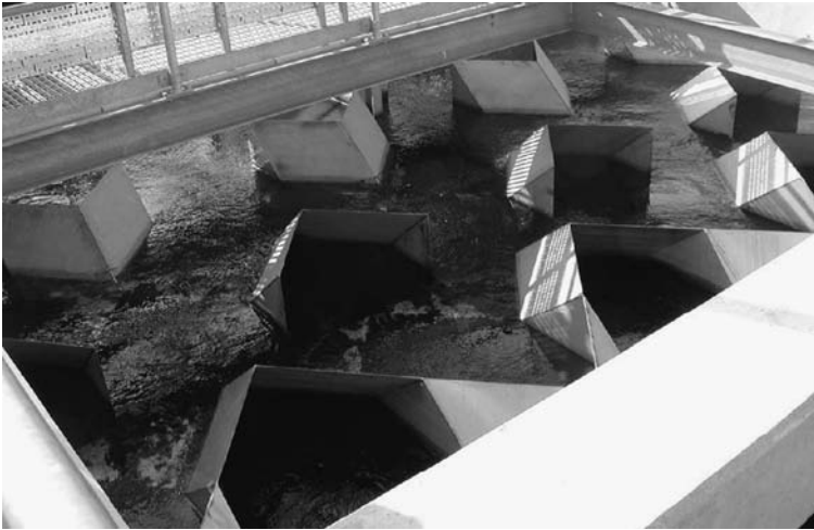
Fig. 4.2 – Hydraulic mixer (courtesy of Sydney Water, Australia)
