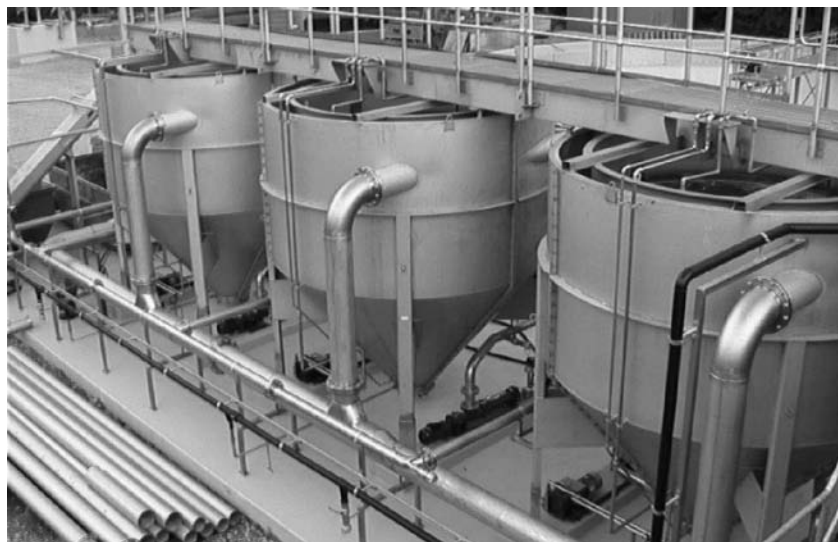
Fig. 3.29 – Circular grit trap (courtesy of Huber, UK)
