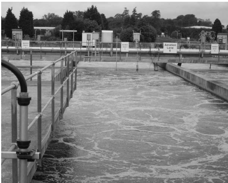
Fig. 6.10 – Activated sludge aeration lane (courtesy of Severn Trent Water, UK)
