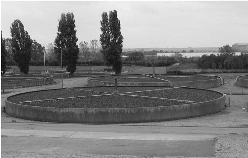
Fig. 6.3 – Trickling filters (courtesy of Anglian Water, UK)
