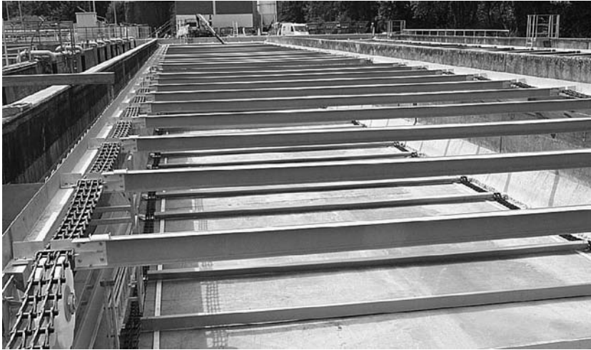
Fig. 3.3 – Horizontal settling tank showing scraper (courtesy of Huber, Germany)
