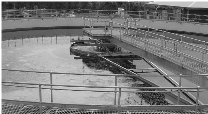
Fig. 3.9 – Secondary clarifier (courtesy of Sydney Water, Australia)
