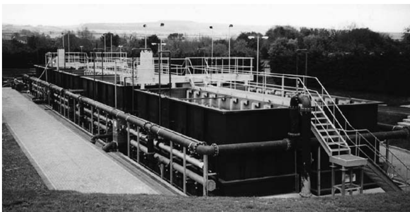
Fig. 7.12 – A submerged membrane bioreactor: microfiltration modules are submerged in the bioreactor tank (courtesy of Aquator Group, UK)
