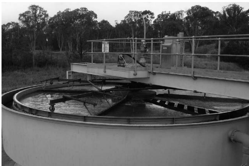
Fig. 3.13 – Dissolved air flotation thickener (courtesy of Sydney Water, Australia)
