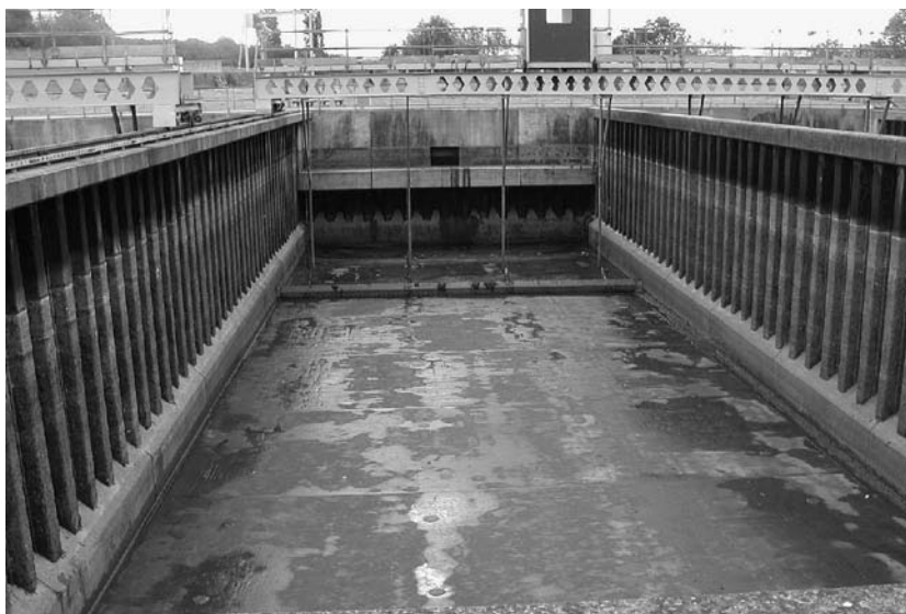
Fig. 3.1 – Wastewater storm tanks (courtesy of Anglian Water, UK)
