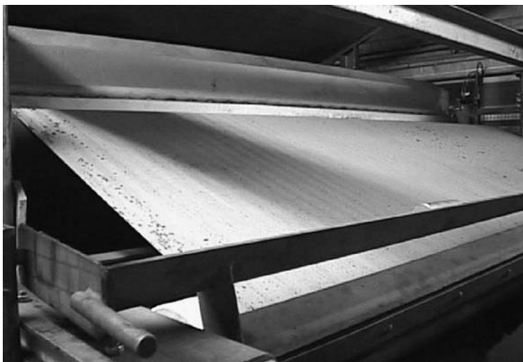
Fig. 8.4 – Belt thickener (courtesy of Anglian Water, UK)
