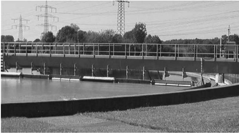
Fig. 3.7 – Skimmer blade on a radial flow settling tank
