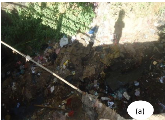
Fig4.5 a) contact of drinking water pipe with solid waste and b) contact of drinking water pipe with liquid wastes
