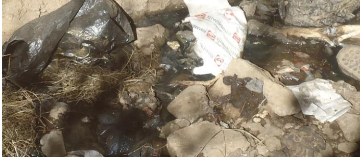
Fig 4.4 drainage lines crammed by stones and other solid wastes
