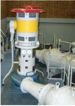
Figure 1.15. Vertical centrifugal pump.
