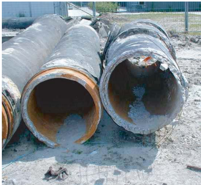
Figure 4.39. Old concrete pipes reinforced with steel net.
