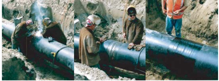
Figure 4.44. Welding of steel pipes.
