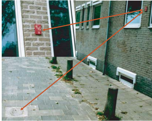
Figure 4.67. Locating underground hydrants (inset shows plate with coordinates).
