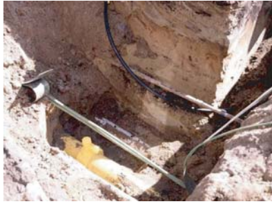
Figure 5.4. Manually excavated trench.
