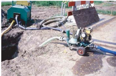
Figure 5.7. Trench dewatering by pumping.
