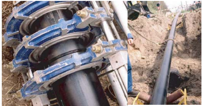
Figure 4.45. Welding and laying of PE pipes.
