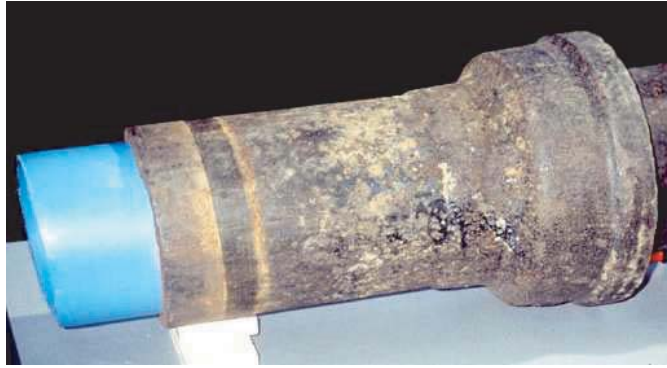
Figure 6.40. Structural relining of an old CI pipe.
