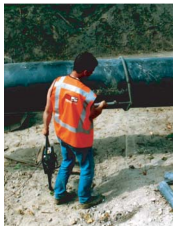
Figure 5.12. Testing of external coating.
