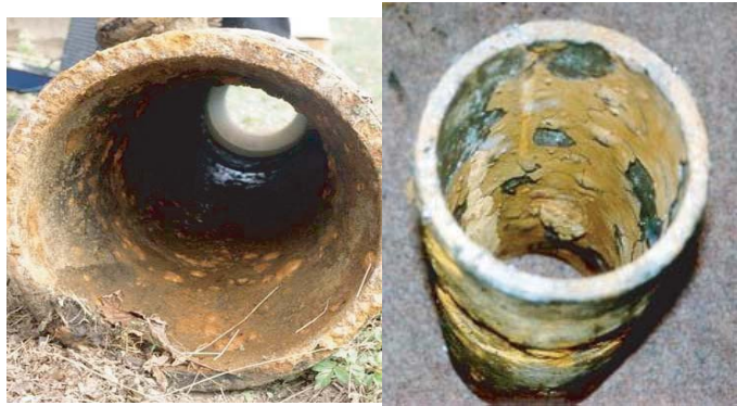
Figure 4.32. Old cast iron pipes.
