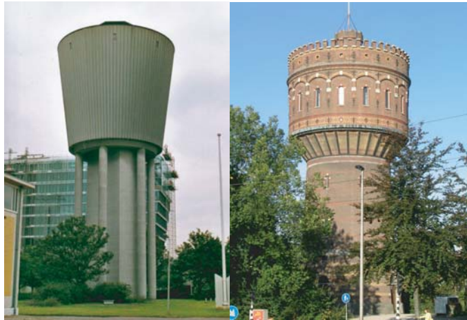
Figure 1.12. Water towers in Amsterdam (still in use) and Delft (no longer in use).
