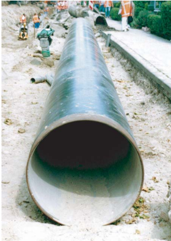
Figure 4.36. Cement lined steel pipe with PE coating.
