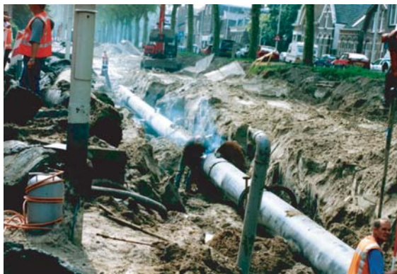
Figure 5.1. Laying of steel pipe.
