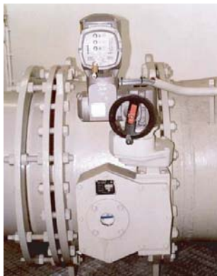
Figure 4.57. Manual and automatic butterfly valve control.
