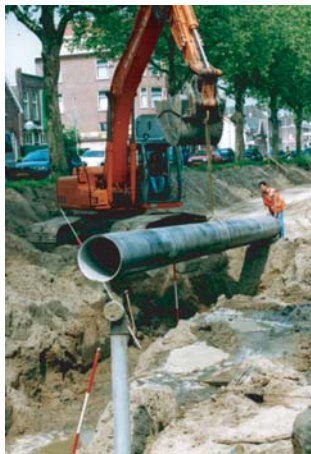
Figure 5.13. Pipe positioning in a trench.
