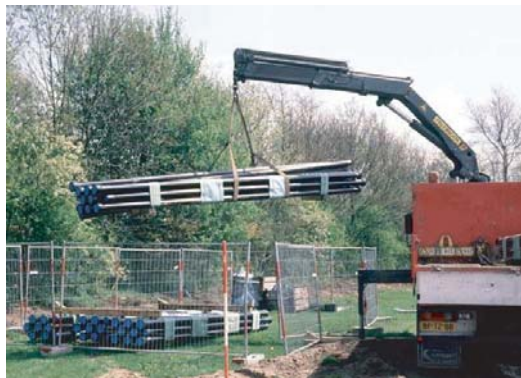
Figure 5.2. Pipe storage on the construction site.
