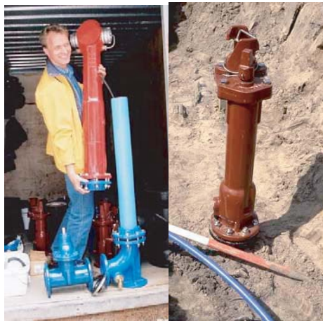
Figure 4.66. Ground level- and underground fire hydrants.
