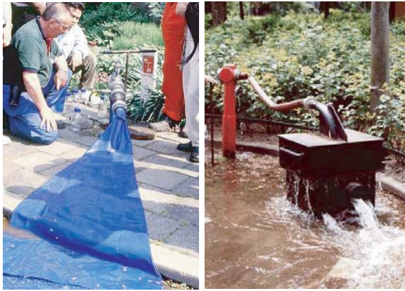
Figure 6.34. Discharge point with dampening of the water jet.
