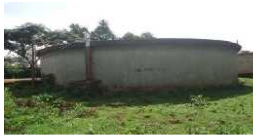
Figure 4.1: Existing service reservoir (source: field observation, March 2016)
