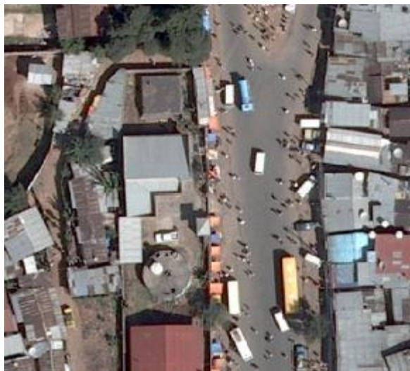
Figure (3.7) Areal view of Entoto Reservoir & Pumping Station (Modified from Google Earth)
