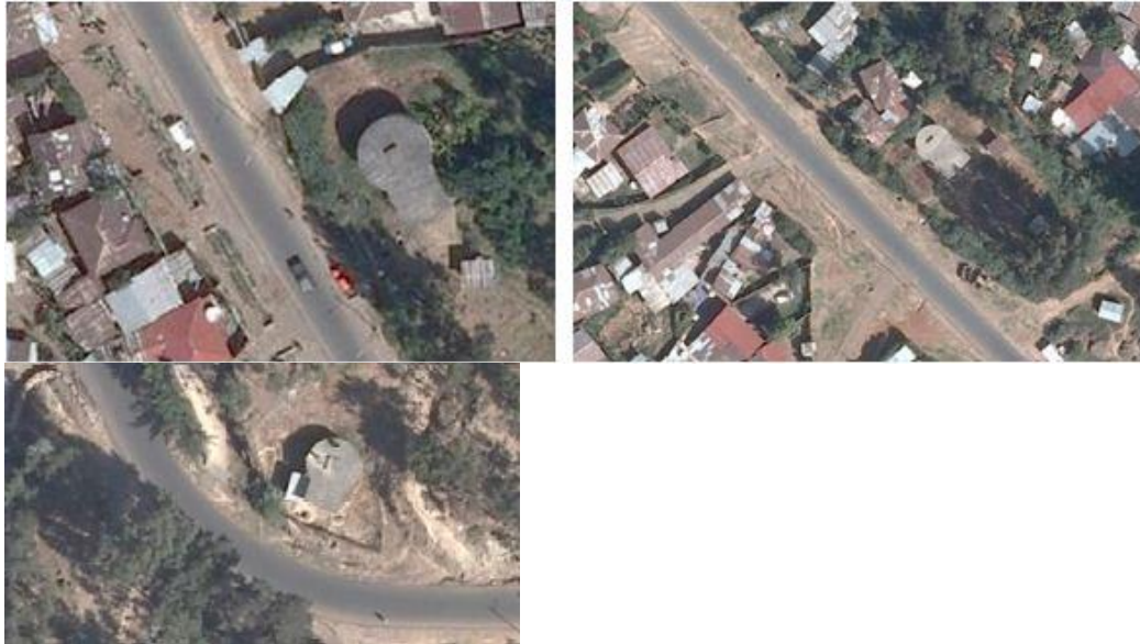
Figure (3.6) Areal view of Upper Entoto Reservoirs (R1, R2 & R3) respectively (Modified from Google Earth)
