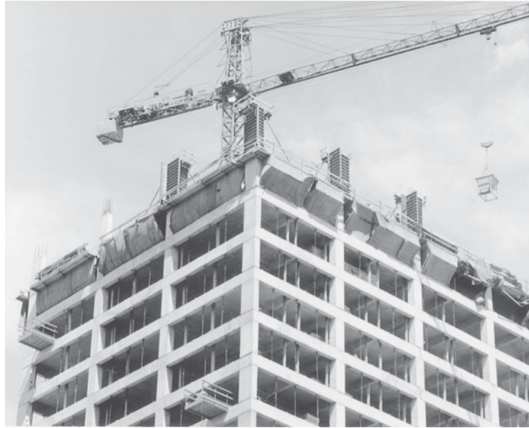
Fig. 10-3 Construction of columns in a tall building. (Photograph courtesy of J. G. MacGregor.)
