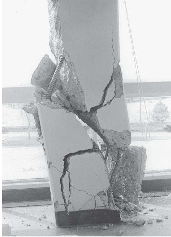
Fig. 6-45 Shear failure in a tied column, 1971 San Fernando earth- quake. (Photograph courtesy of U.S. National Bureau of Standards.)
