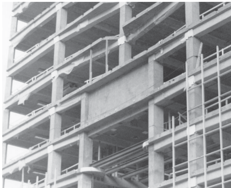
Fig. 17-25 Single-span deep beam. (Photograph courtesy of J. G. MacGregor.)
