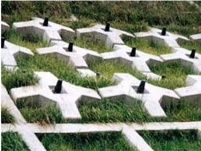
Ground Anchor Work
