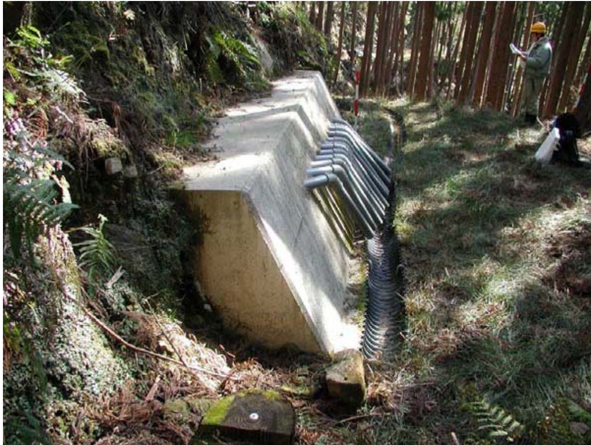
Horizontal Drainage Work
