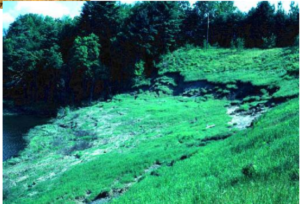
This landslide was triggered by heavy rainfall
