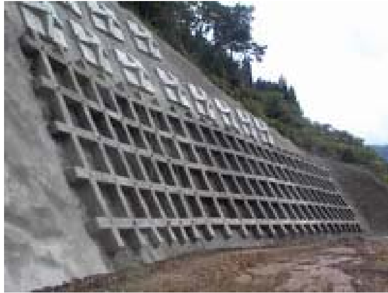
Rock Bolt Work + Frame Work
