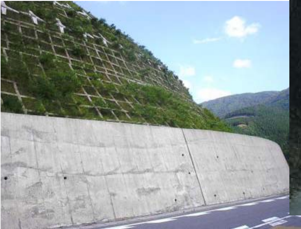
RC Retaining Wall
