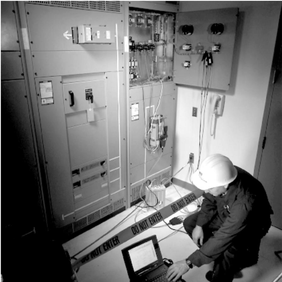
**FIGURE 9.13** Proper personal protective equipment (PPE), which is essential to performing power quality instrument setup and testing. The photograph shows the use of fire-retardant clothing, safety hat, and shoes. Safety glasses must be worn while connecting instrument probes to the test point. The test location shown here is properly barricaded to prevent unauthorized persons from entering the area.
