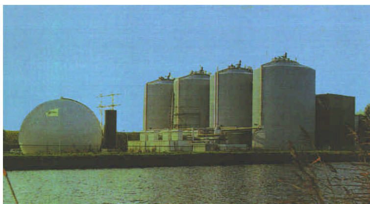
Figure 2.9 Anaerobic digestion for CHP production Vagron Groningen plant
