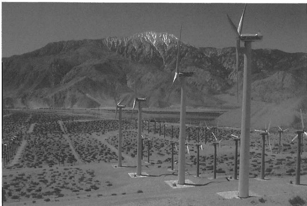
Figure 8.3 A wind farm in San Geronio Pass, Palm Springs, California (Reproduced by permission of Henry Dupont)
