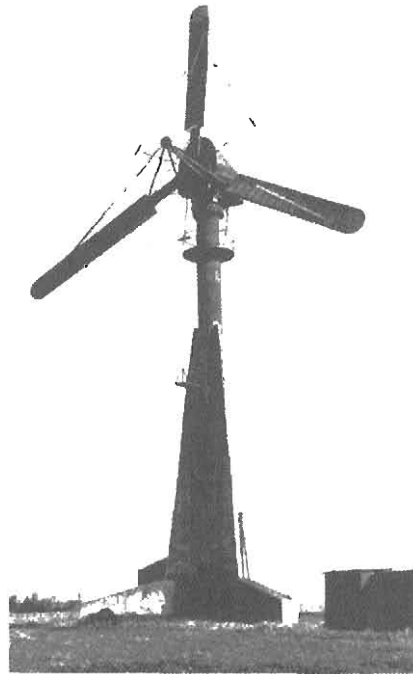
Figure 1.12 Danish Gedser wind turbine. Reproduced by permission of Danish Wind Turbine Manufacturers
