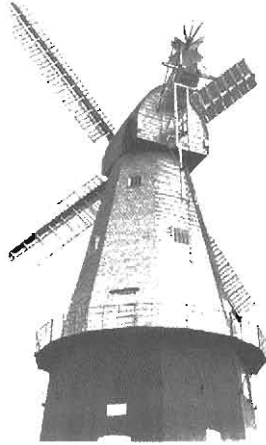
Figure 1.8 European smock mill (Hills, 1994). Reproduced by permission of Cambridge University Press
