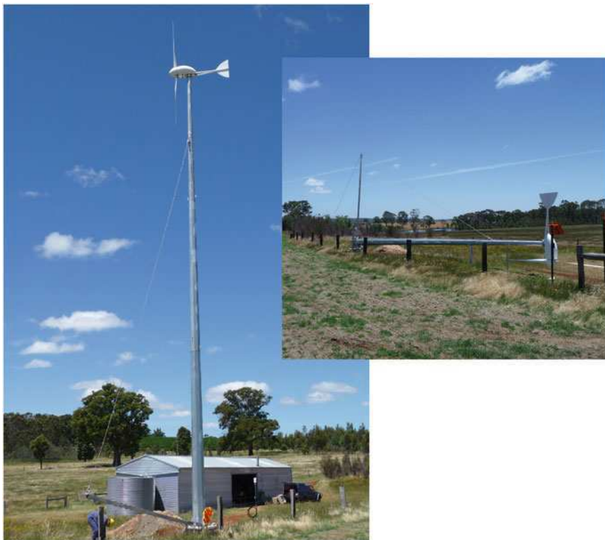
Fig. 10.2 The Aerogenesis 5 kW turbine on its 18 m monopole tower. The gin pole for raising and lowering is attached near the base. The right side photo shows the turbine before being raised (photos from Paul Peterson)
