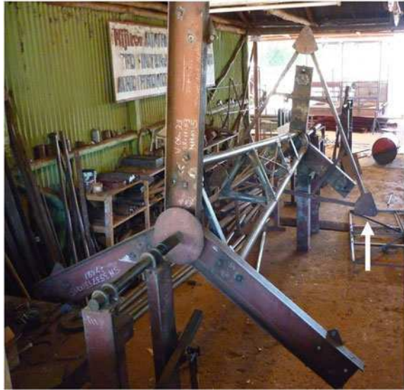
Fig. 10.8 Jig to make 3 m long sections of a tubular lattice tower at Kijito Windpower, Kenya. The top section of a tower is in the jig and one of the three base plates for the bottom section is shown by the white arrow
