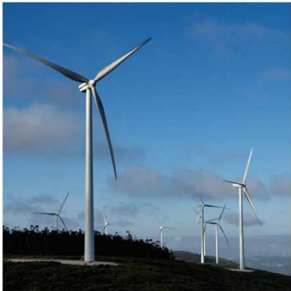
Fig. 1.3 Vestas 2 MW V80 wind turbines
