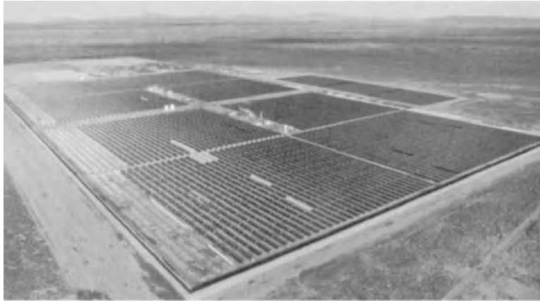
Figure 17.3.1 Aerial view of SEGS III, IV, and V, three of the Luz plants located on the Mojave Desert of southern California. Photo courtesy of Luz International, Inc.
