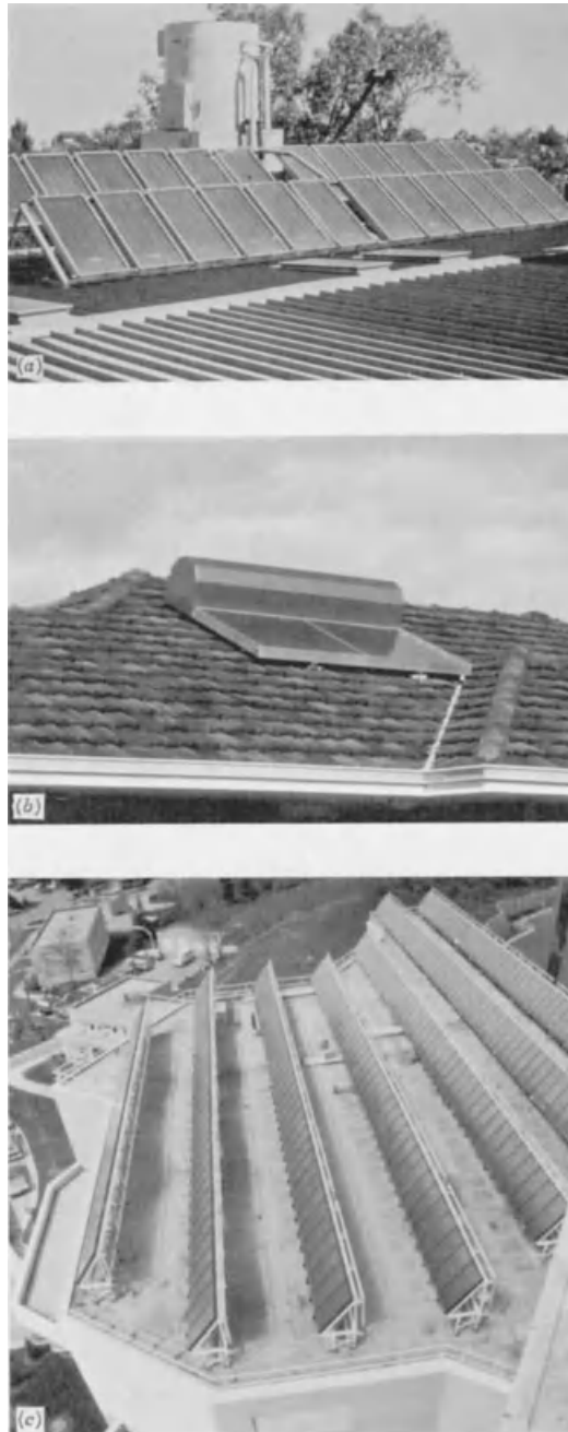
Figure 12.1.2 Solar water heaters. (a) Natural-circulation system on hostel, Griffith, Australia. Photo courtesy of CSIRO. (b) Domestic system, with coupled tank and collector, Perth, Australia. (c) Hospital service hot-water system, Madison, WI. Photo courtesy of Affiliated Engineers, Inc. (d) Collectors for a domestic system, Madison, WI.
