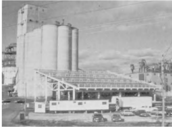
Figure 16.4.2 The 1200-m 2 air heating collector array at the Gold Kist soybean plant at Decatur, AL. Courtesy of Solaron Co.
