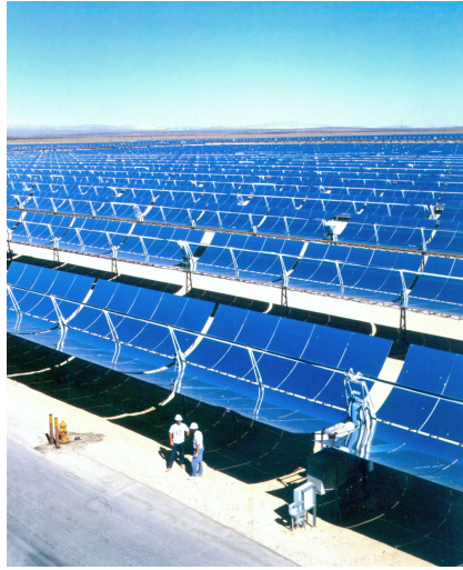
Fig. 10.12. Solar trough collectors at Kramer Junction (courtesy of DOE/NREL).
