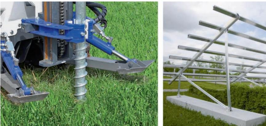
**Figure 6.27** Alternative ground fixings: Screwed foundation as well as concrete heavy-load foundations (photos: Krinner Schraubfundamente GmbH, Schletter GmbH)
