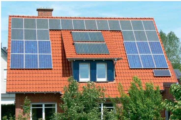
**Figure 6.32** On-roof system on a private house: There should be at least a row of tiles spacing at the side in order to reduce attack possibilities for the wind
