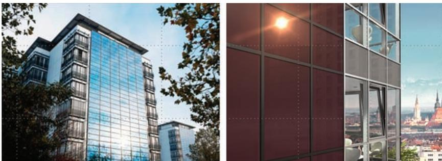
**Figure 6.35** View of two façade installations: *Left*: a 50 kWp system of polycrystalline modules in Freiburg, Germany (source: Solarfabrik AG). *Right*: cold façade Prosol TF+ of a-Si modules (source: Schüco International KG)
