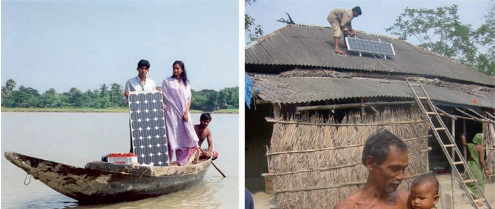
**Figure 7.36** Photos of solar home systems in Bangladesh: Arrival of the components by river and installation of the plant on a hut (photos: Grameen Shakti; Microenergy International)
