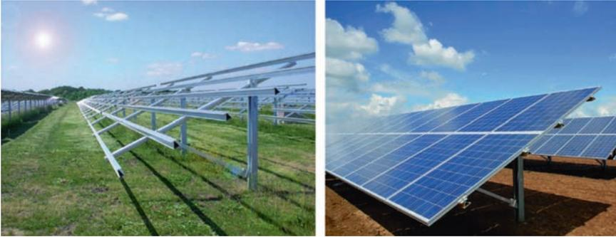
**Figure 6.26** Typical construction of an open air plant: Galvanized steel posts are rammed into the ground and serve as the base for the module panel support. (photo: Schletter GmbH)
