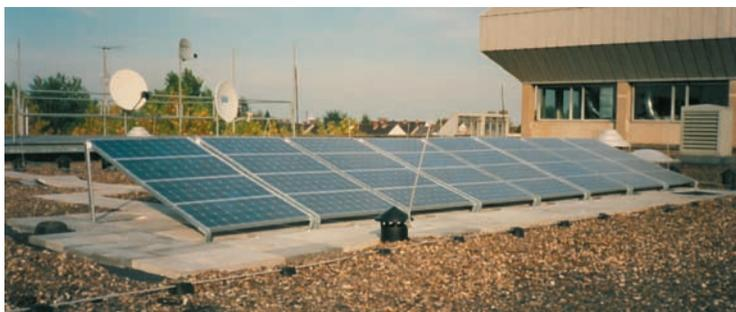
**Figure 6.29** Photovoltaic plant at the Münster University of Applied Sciences from 1994: The aluminum support structure is held down by means of flagstones (photo: W. Göbel)
