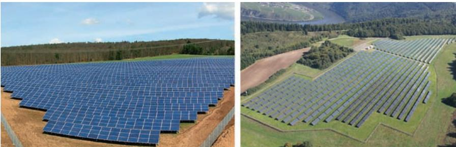
**Figure 6.25** View of two solar parks: *Left*: Citizen solar park Hofbieber-Traisbach with 1.3 MWp of polycrystalline modules (photo: IBC SOLAR AG). *Right*: 3.5 MWp solar park at Mehring on the Moselle with CdTe modules (photo: juwi Solar GmbH)
