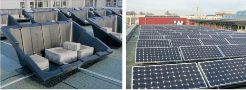
**Figure 6.30** Flat roof system on the roof of the Münster University of Applied Sciences of the year 2008: The modules are placed in plastic tubs that are again weighed down by paving stones
