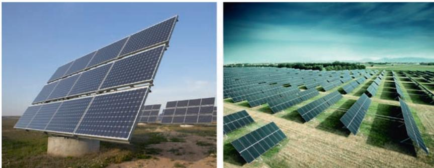
**Figure 6.28** Tracked open air plants: Dual-axis Solon-Mover as well as single-axis system with horizontal axis (photos: Urnato © SOLON)
