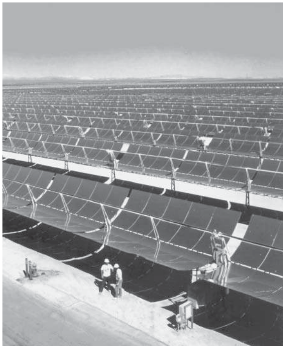
Figure 17.3.3 (a) SEGS collector fields.
