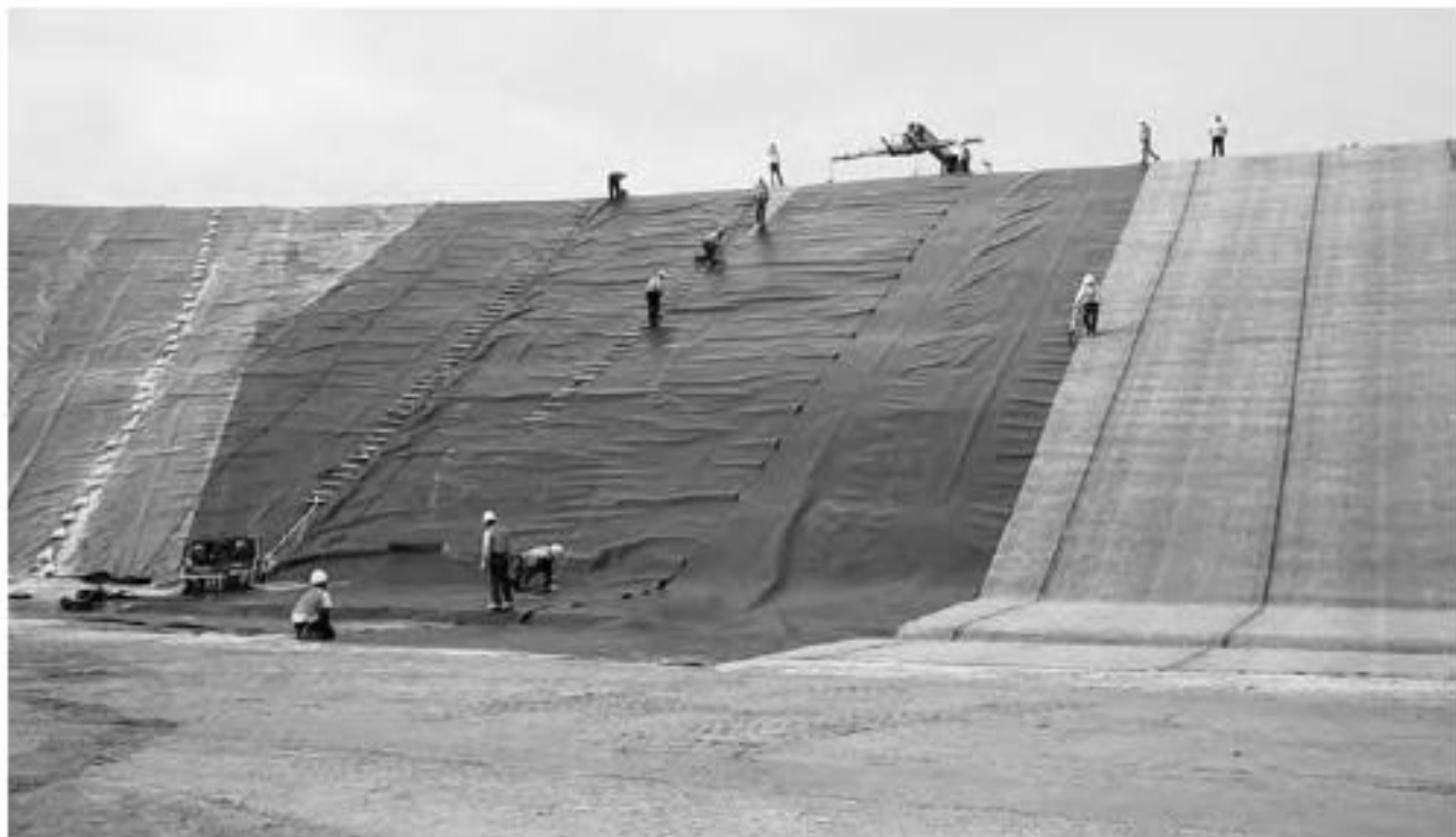
Figure 4-10 Synthetic liner on slope, ready for earth cover. (Courtesy William A. Worrell)
