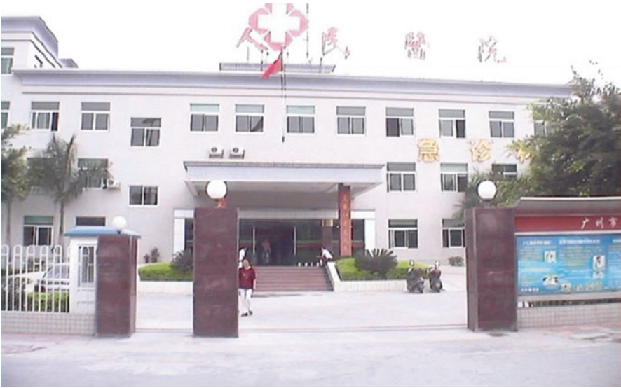
Fig. 4.4 The hospital of Long Village
