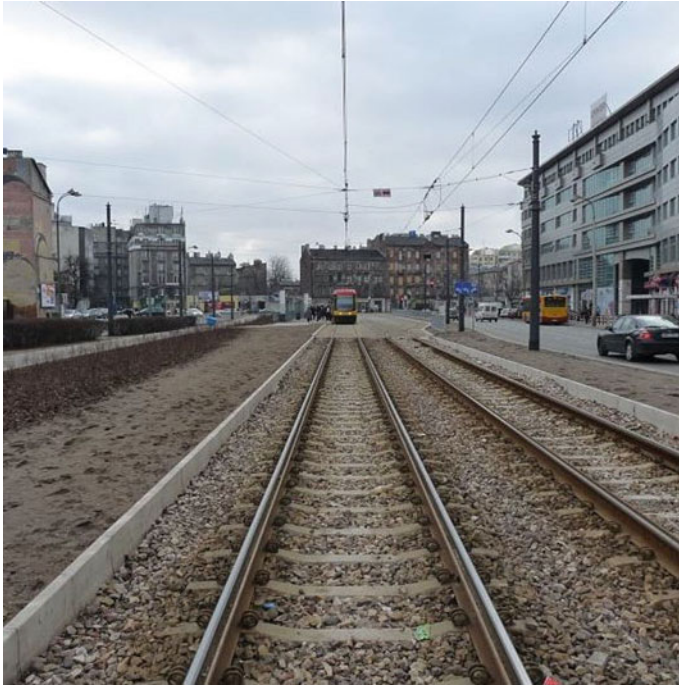
Fig. 8.8 One of the modifications of the rail fastening of SB-3 type used for tram tracks in Warsaw (2012) ( http://www.garnek.pl/lumiks/20076979/tor-tramwajowy-1435mm-lok# )
