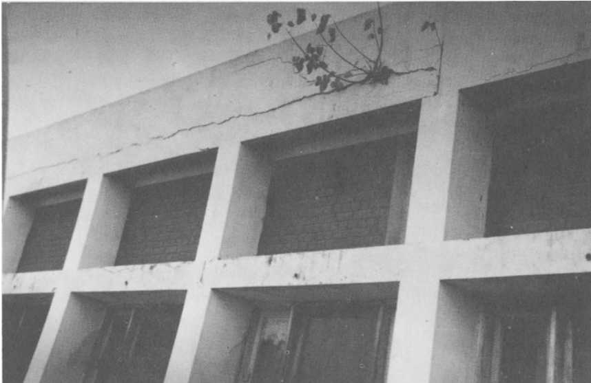
Figure 8.6 Plant damage to a building.
