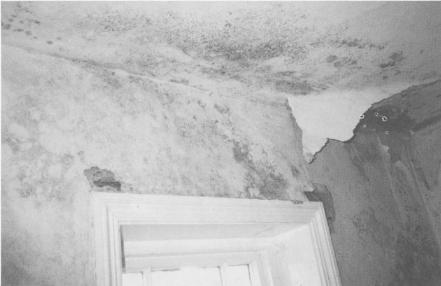
Figure 8.3 Mould growth in buildings.
