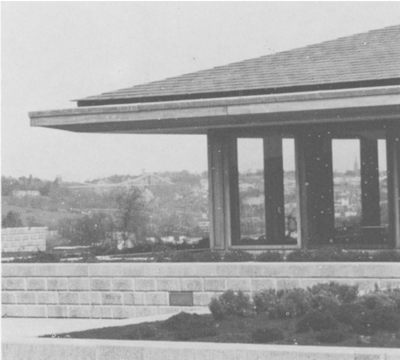
Figure 4.3 (above and right) At the offices for the SW Regional Headquarters of the CEBG in Bristol, the building fabric is used to assist cooling in summer. During the night, fresh air is passed through the hollow concrete floors thus cooling the structure. Daytime air passed through the same routes is then cooled by the concrete structure before it is distributed to the offices. When combined with reducing waste heat from lights and suitable shading of windows, it ensures that the office temperature can be maintained without the need for mechanical chilling. In winter, waste heat from machinery, lights and computers is stored in the staff swimming pool and is extracted by heat pumps for the hot water system. (Courtesy of Arup Associates, Architects & Engineers & Quantity Surveyors.)
