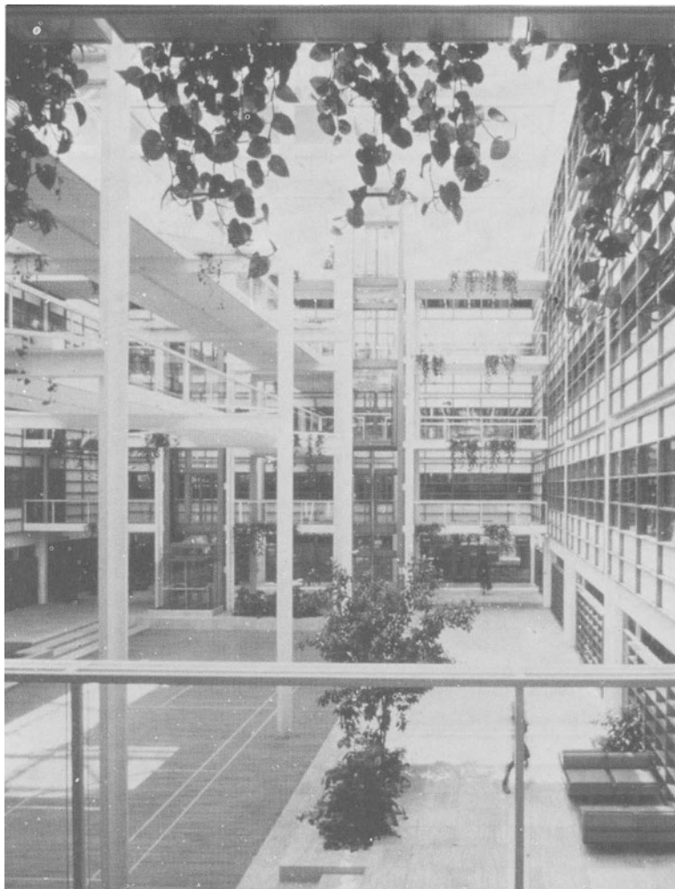
Figure 4.6 (above and right) Gateway 2 at Basingstoke is an office building with a floor area of about 16 000 m 2 where the offices are planned around a central atrium. The offices have views to the atrium as well as to the outside. As well as being an amenity the atrium also acts as a natural chimney drawing fresh air across the offices and out through opening ventilators in the roof. As a result, it is possible to ventilate naturally a building which would normally have required air conditioning. The occupants can control the degree of ventilation simply by opening or closing their office windows. By enclosing an internal courtyard, heat gains and losses are also reduced. (Courtesy of Arup Associates, Architects & Engineers & Quantity Surveyors.)
