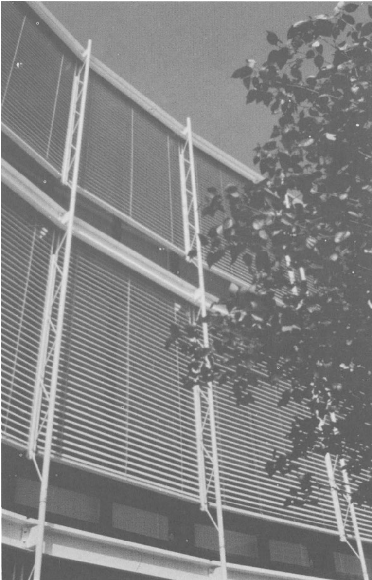
Figure 4.8 (above and right) External sun shading can prevent the sun penetrating into a building and thereby drastically reduce the radiant heat gain. By careful design it should protect the interior from summer sunshine while ensuring good outlook for people using the building. (Courtesy of Arup Associates, Architects & Engineers & Quantity Surveyors.)
