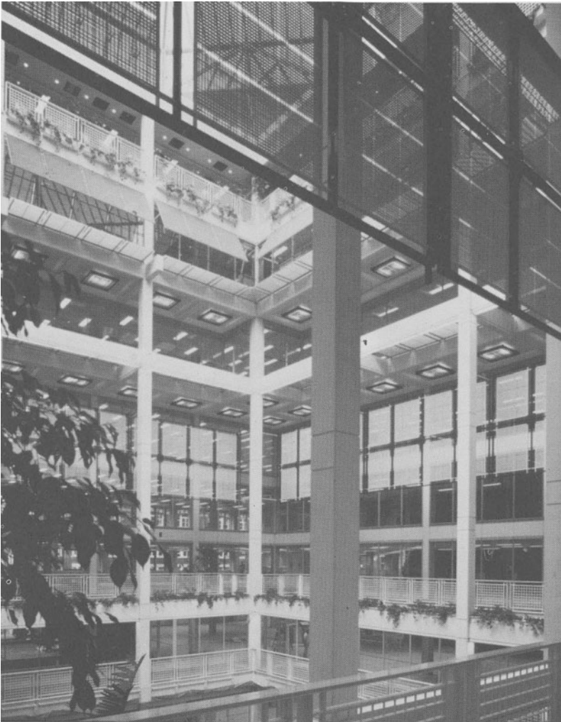
Figure 4.2 (above and right) Direct sunlight can strike the glazed walls of offices through a top-lit atrium and it is important to design internal screens which are appropriately located to protect work areas from glare and unnecessary heat gain. (Courtesy of Arup Associates, Architects & Engineers & Quantity Surveyors.)
